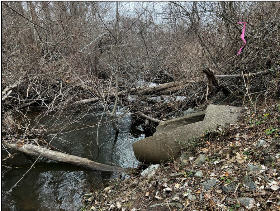
Photo 1: View of stormwater discharge pipe outlet into river near wetland flag #10.
