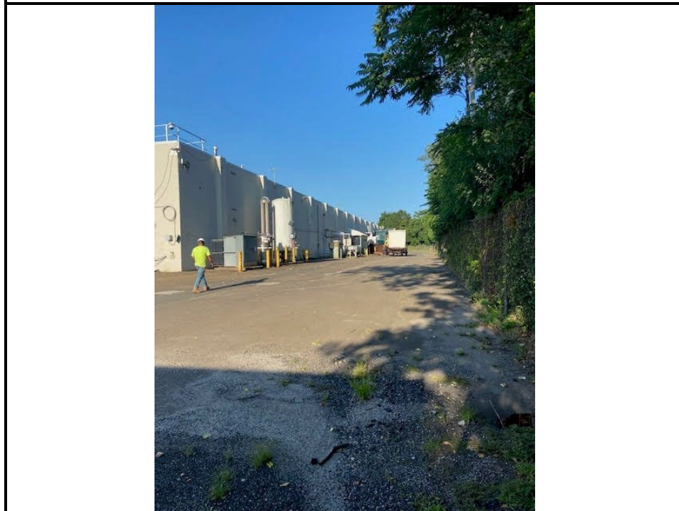
Photo 10: View of Interconnection Corridor facing West
