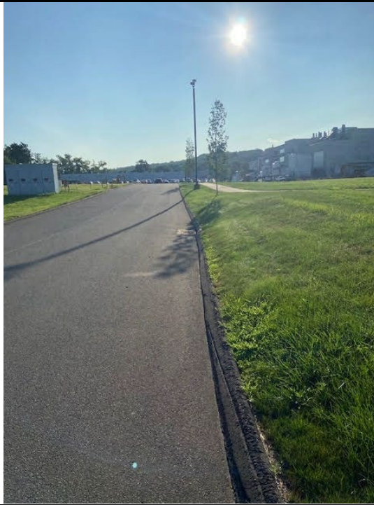
Photo 1: View of Site Access facing East
