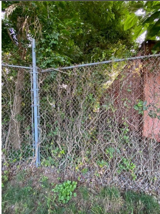
Photo 12: View of Property Line facing East
