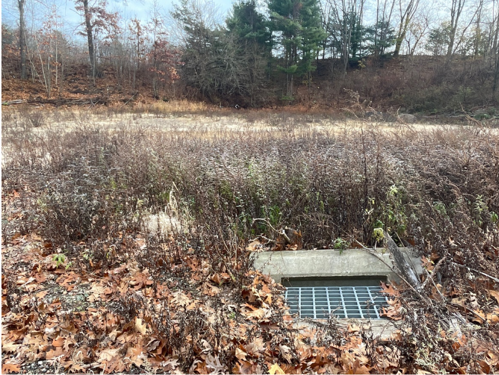
Storm drain connected to wetland W-MFT-1
