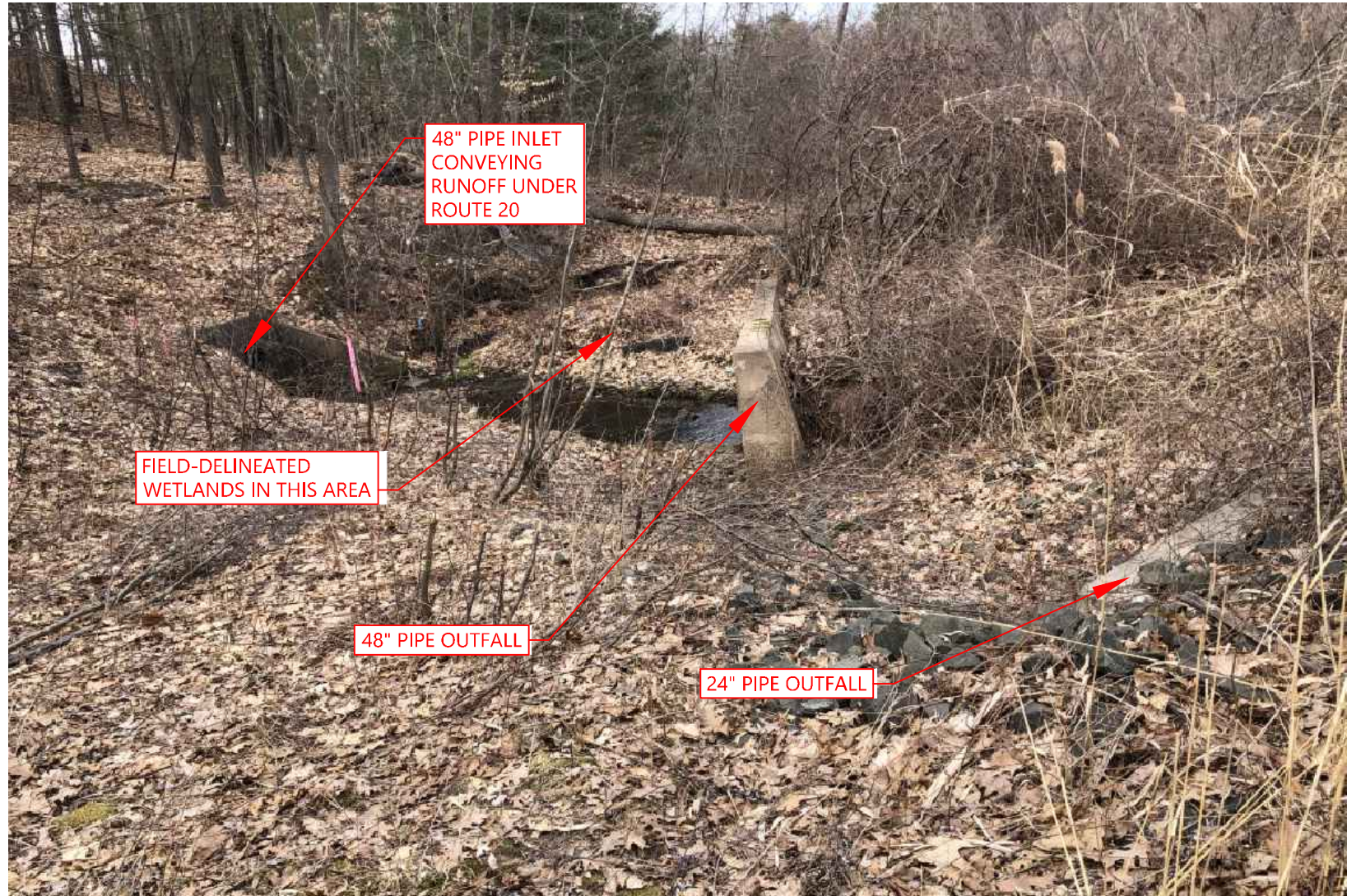
Photo 7 Wetlands and Pipe Outfalls
