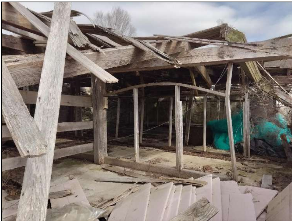
Photo 22. Overview of barn foundation interior. Photo facing to the northeast.
