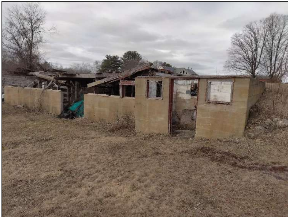
Photo 20. Overview of barn foundation. Photo facing to the northwest.
