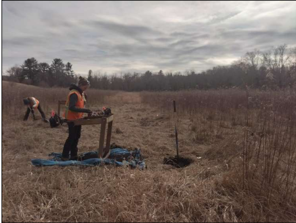
Photo 7. Overview of excavations within SA-3. Photo facing to the west.
