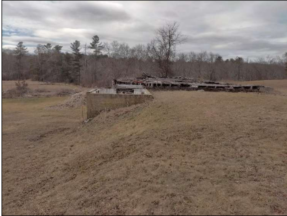
Photo 19. Overview of barn foundation. Photo facing to the west.
