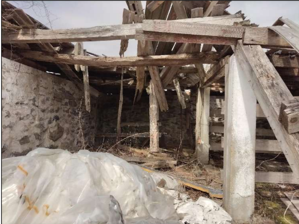
Photo 21. Overview of barn foundation interior. Photo facing to the north.
