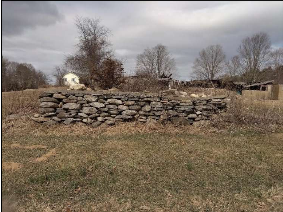
Photo 15. Overview of Barn foundation. Photo facing to the north.
