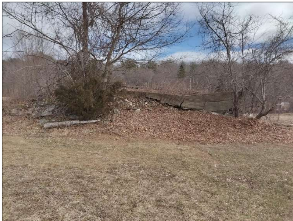
Photo 18. Overview of barn foundation. Photo facing to the east.
