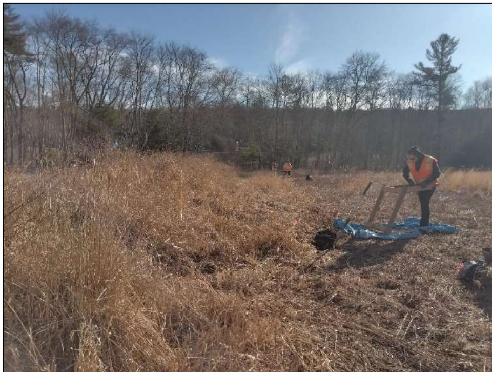
Photo 2. Overview photo of excavation within SA-2. Photo facing to the East.
