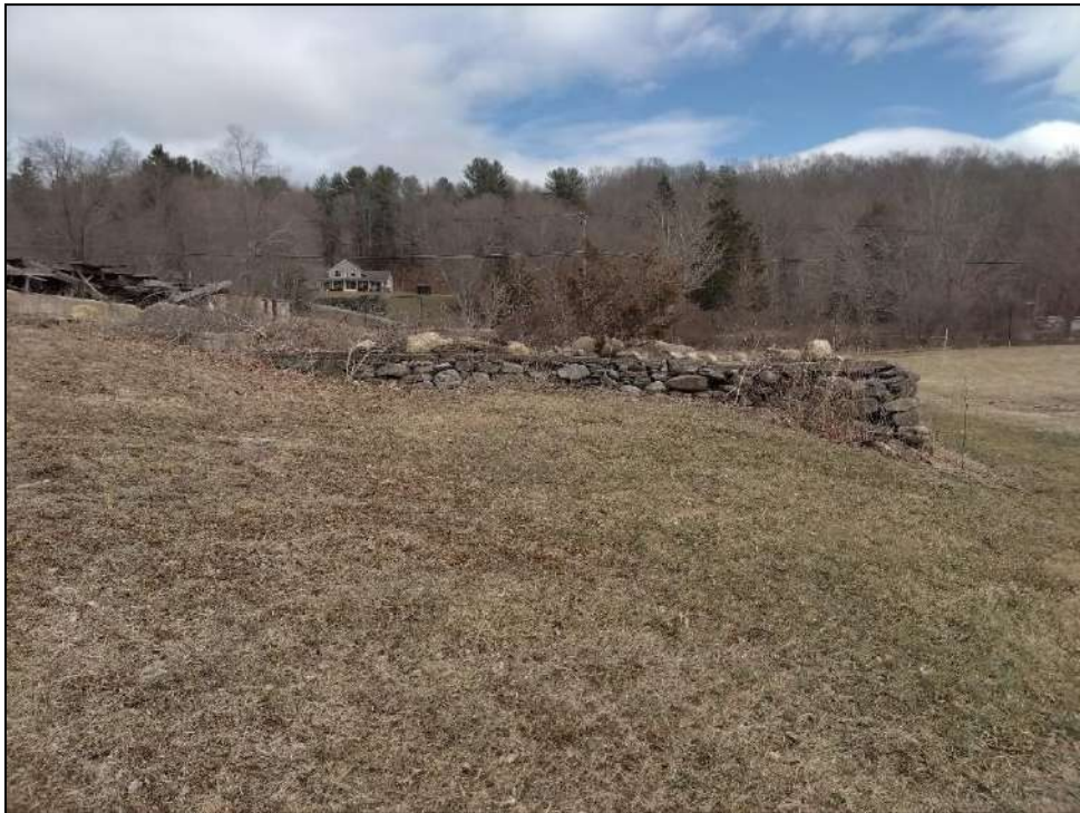
Photo 16. Overview of barn foundation. Photo facing to the east.
