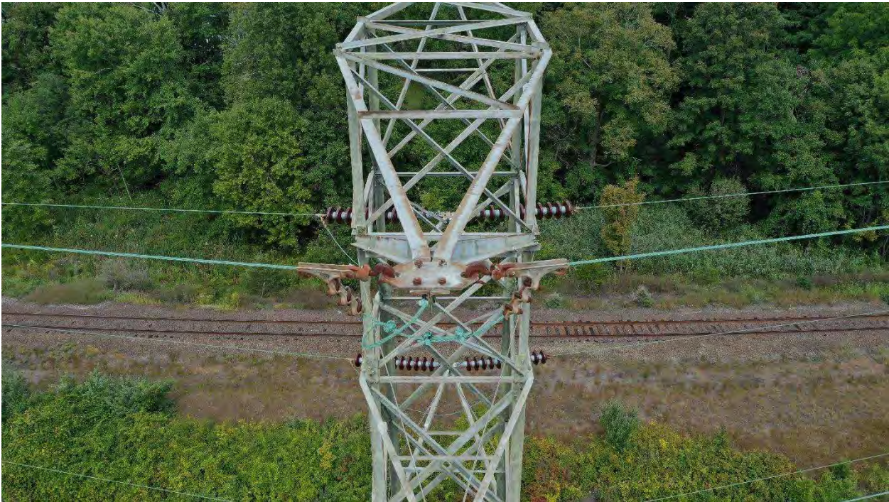
Structure 4647: rusting lattice tower members
