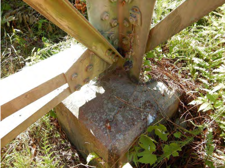
Structure 4602: rusting hardware
