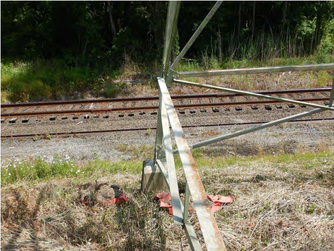
Structure 4647: rusting lattice tower members
