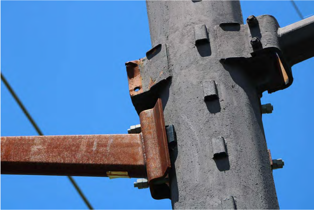
Structure 4602: rusting hardware
