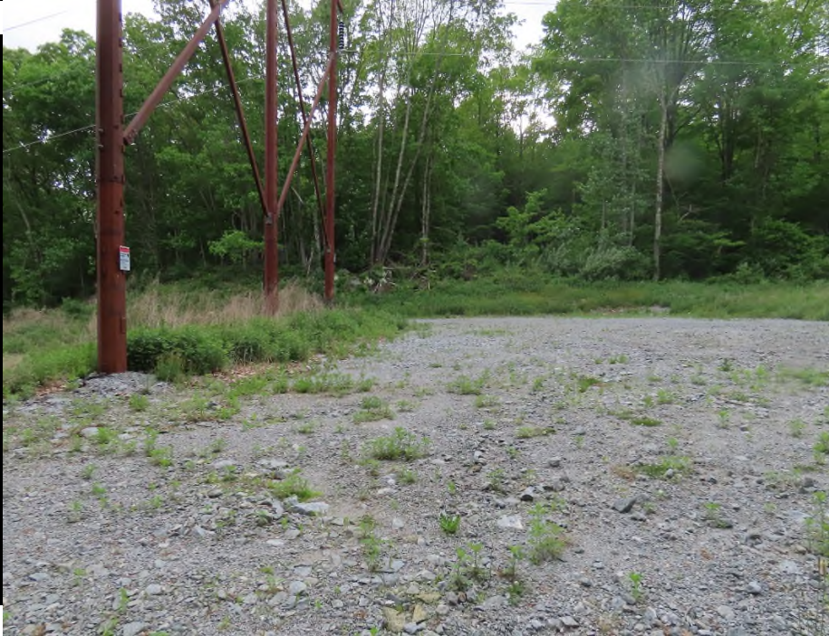
Photo 3-3: W. view of forest edge from large, sparse gravel pad N. of Pole 7786.
