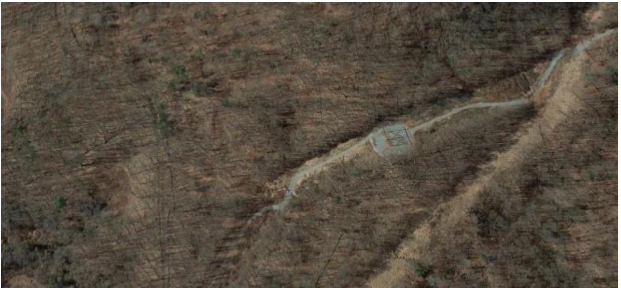
Photo of site 7786 after construction.
