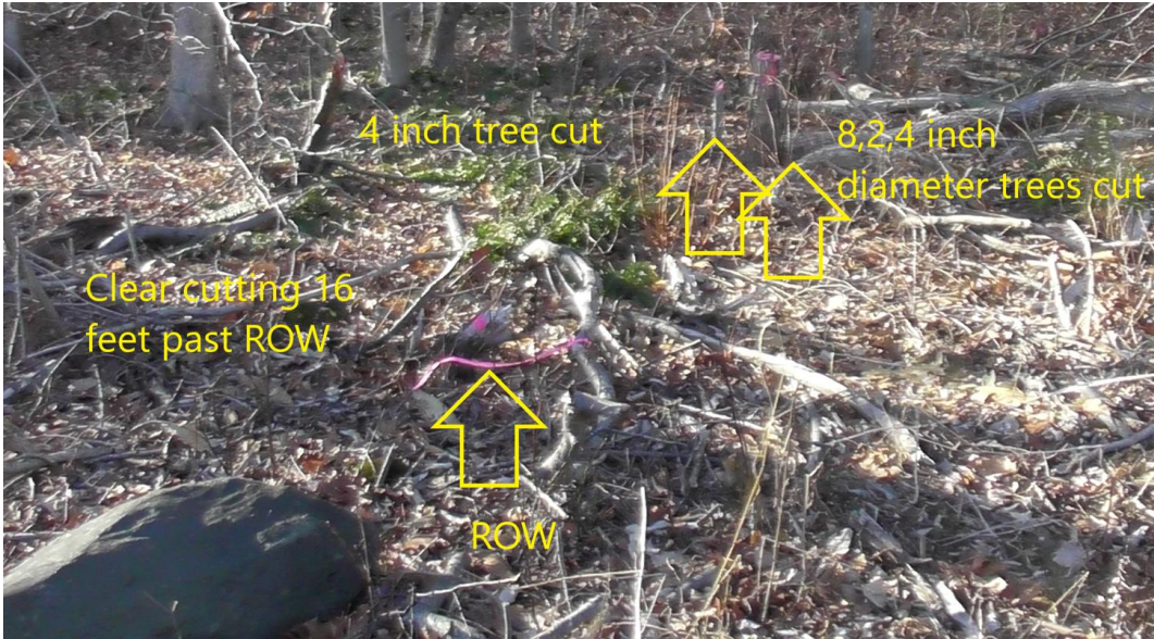
Same area, 11-inch diameter tree cut down 16 feet beyond the easement.
