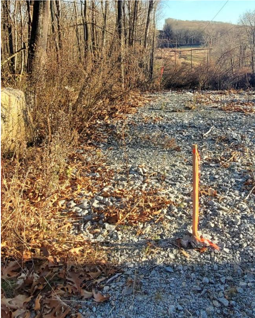
This photo shows the Eversource placed stake that defines the ROW limit at site 7785. Note the extensive filling and grading outside of the easement.
