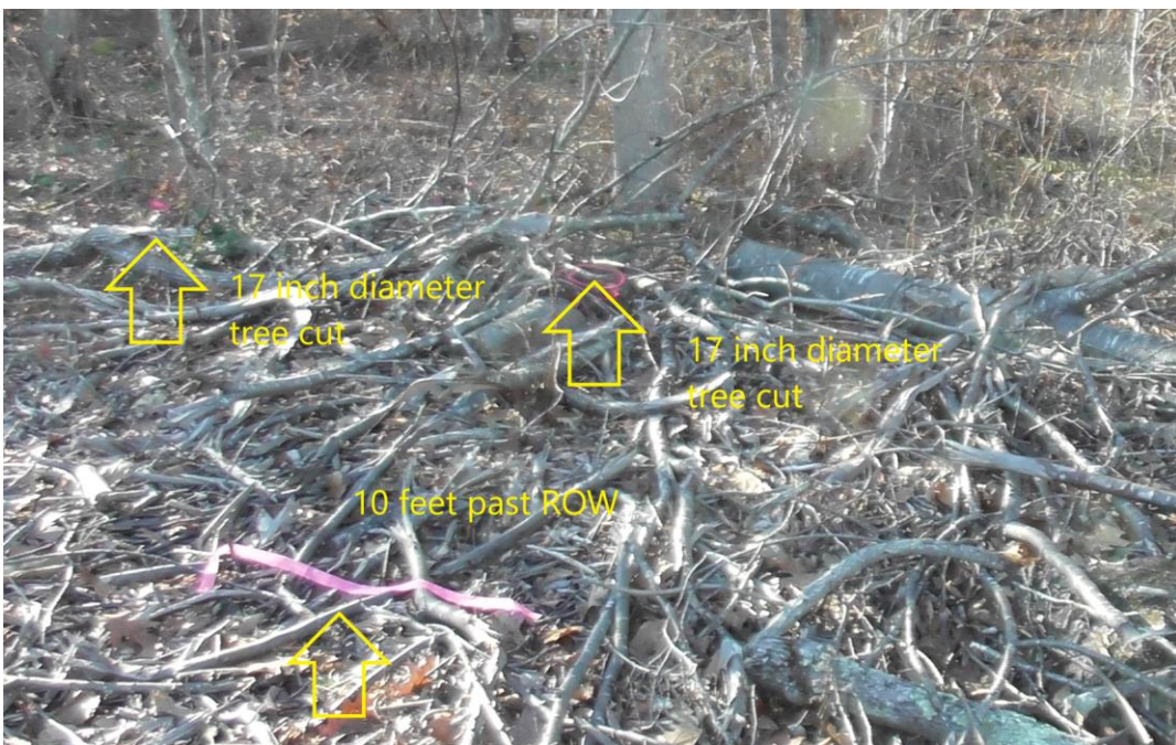
And this, showing a 17-inch diameter trees cut down 10 feet beyond the easement.
