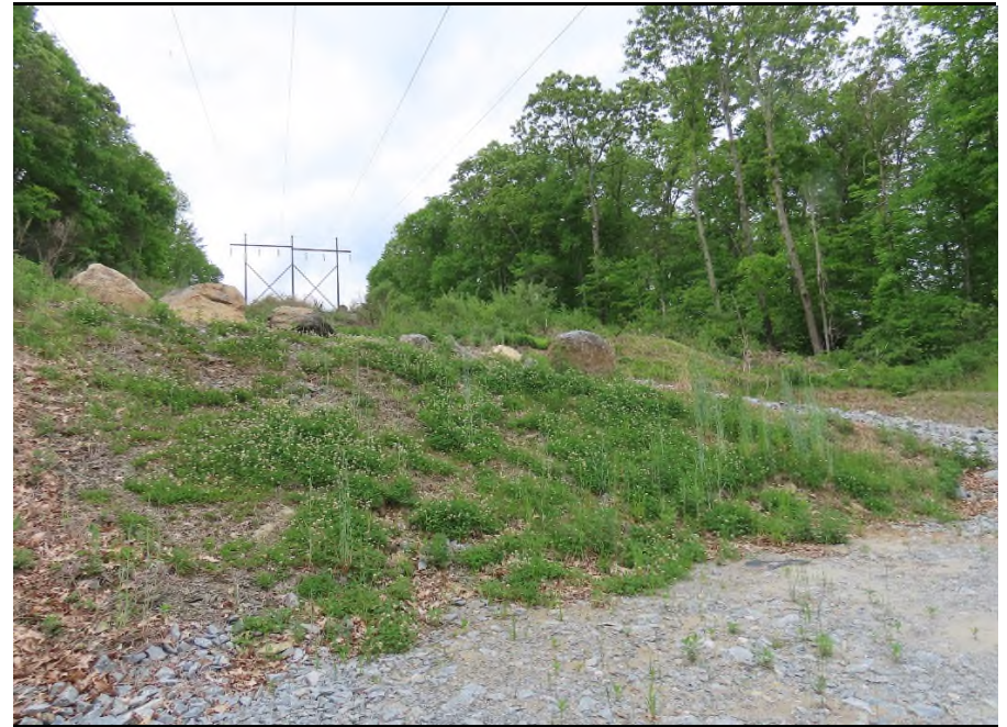
Photo 3-2. N view to Pole 7786. On cut slope clovers sprouted from seed mix
