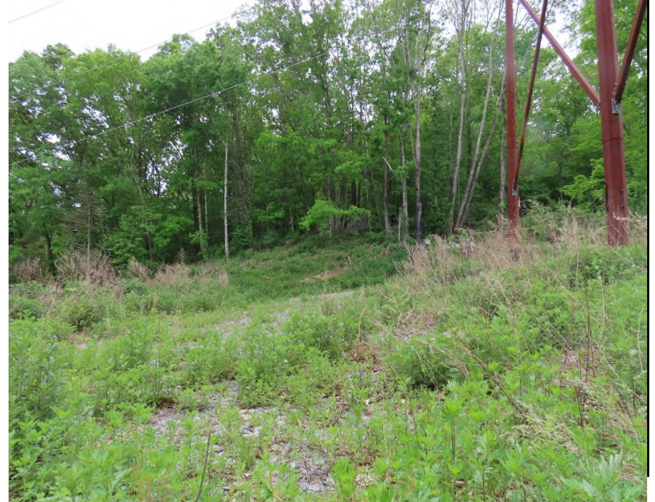
Photo 3-4: Westerly view. Sparse compacted ground S. of pad at Pole 7786.
