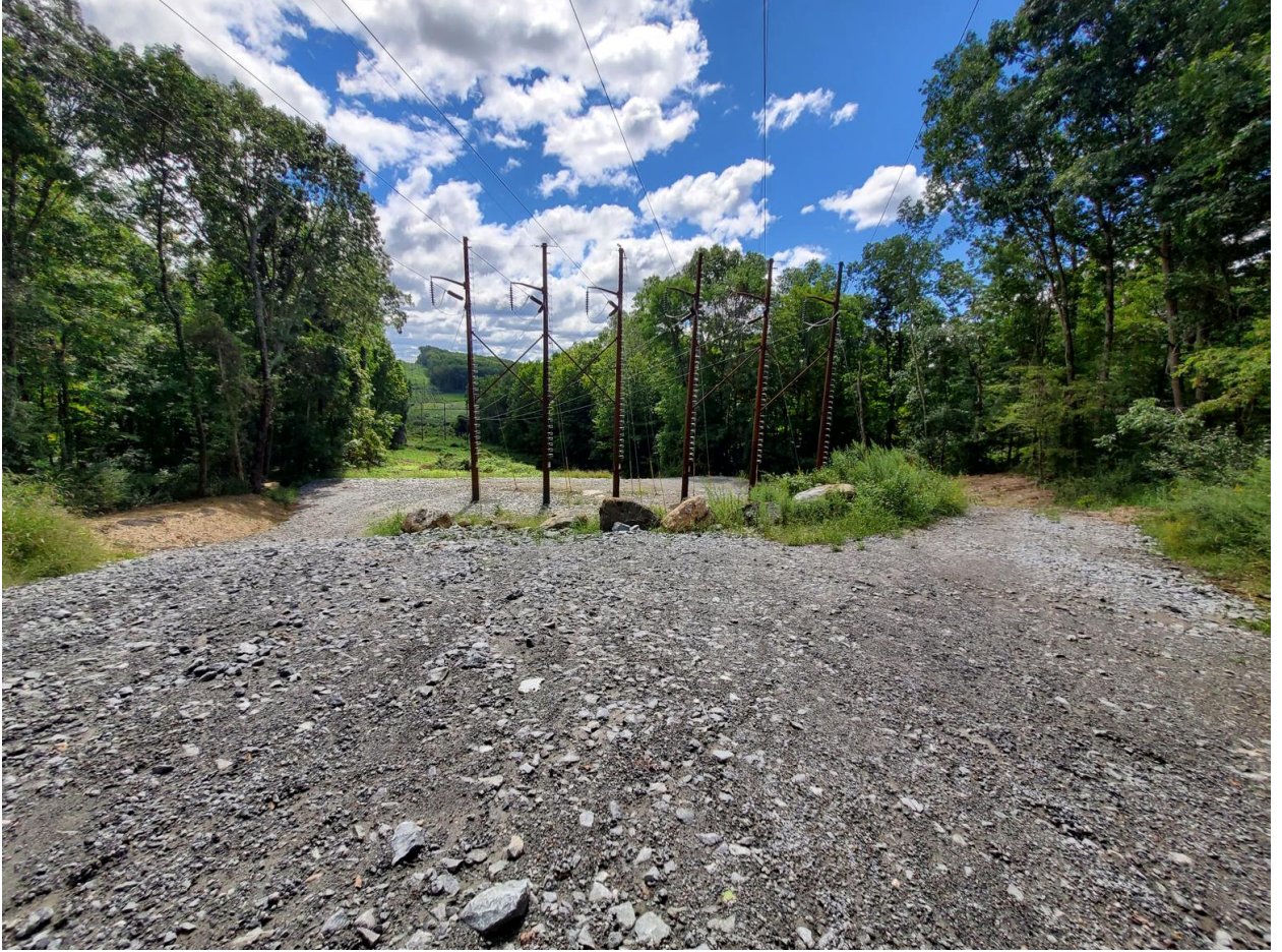
And more erosion.
