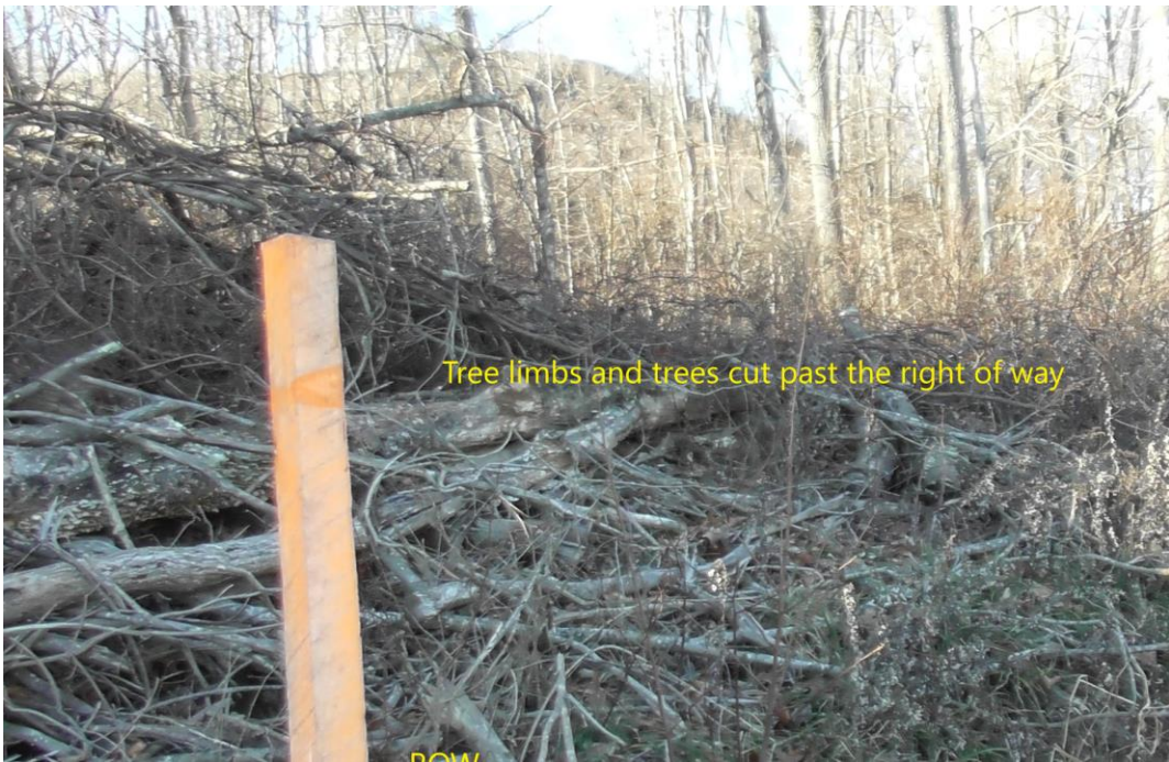
At site 7786 on the west side is this evidence of all the trees cut down outside the easement and the debris left.
