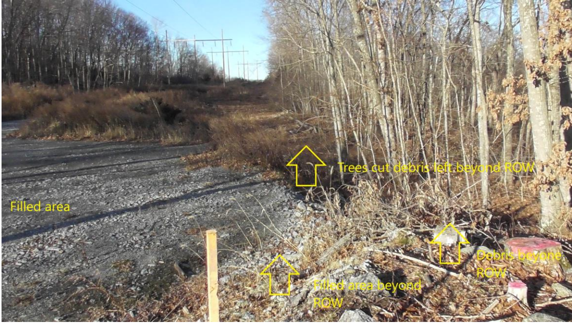
This photo depicts crushed rock fill deposited outside the easement and the debris left near site 7786.
