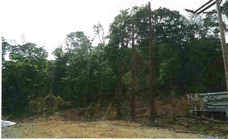
Str 7785 during construction – taken June 9, 2021
