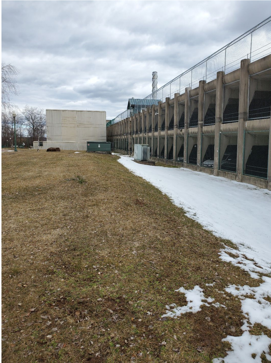
Looking east from Facility location; water cooling tower and Energy Center stack in background
