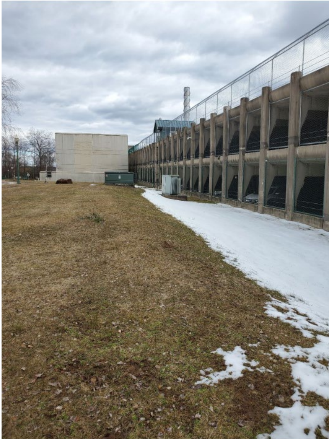
Looking east from Facility location; water cooling tower and Energy Center stack in background
