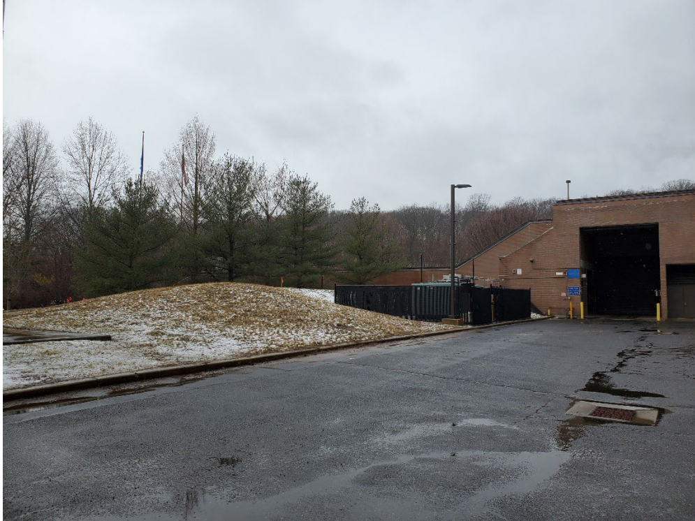
Looking toward Facility area
