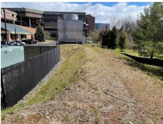
Image 3 – Left of Fuel Cell Install Area
