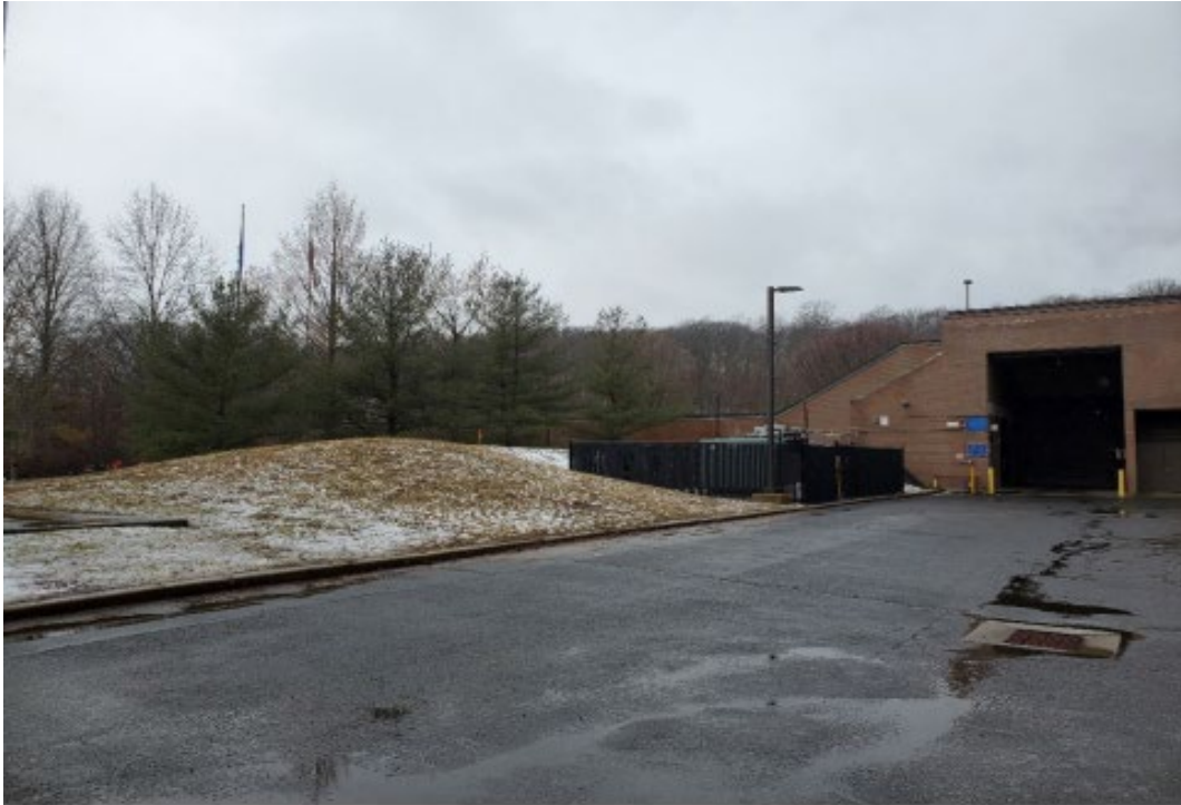
Looking toward Facility area
