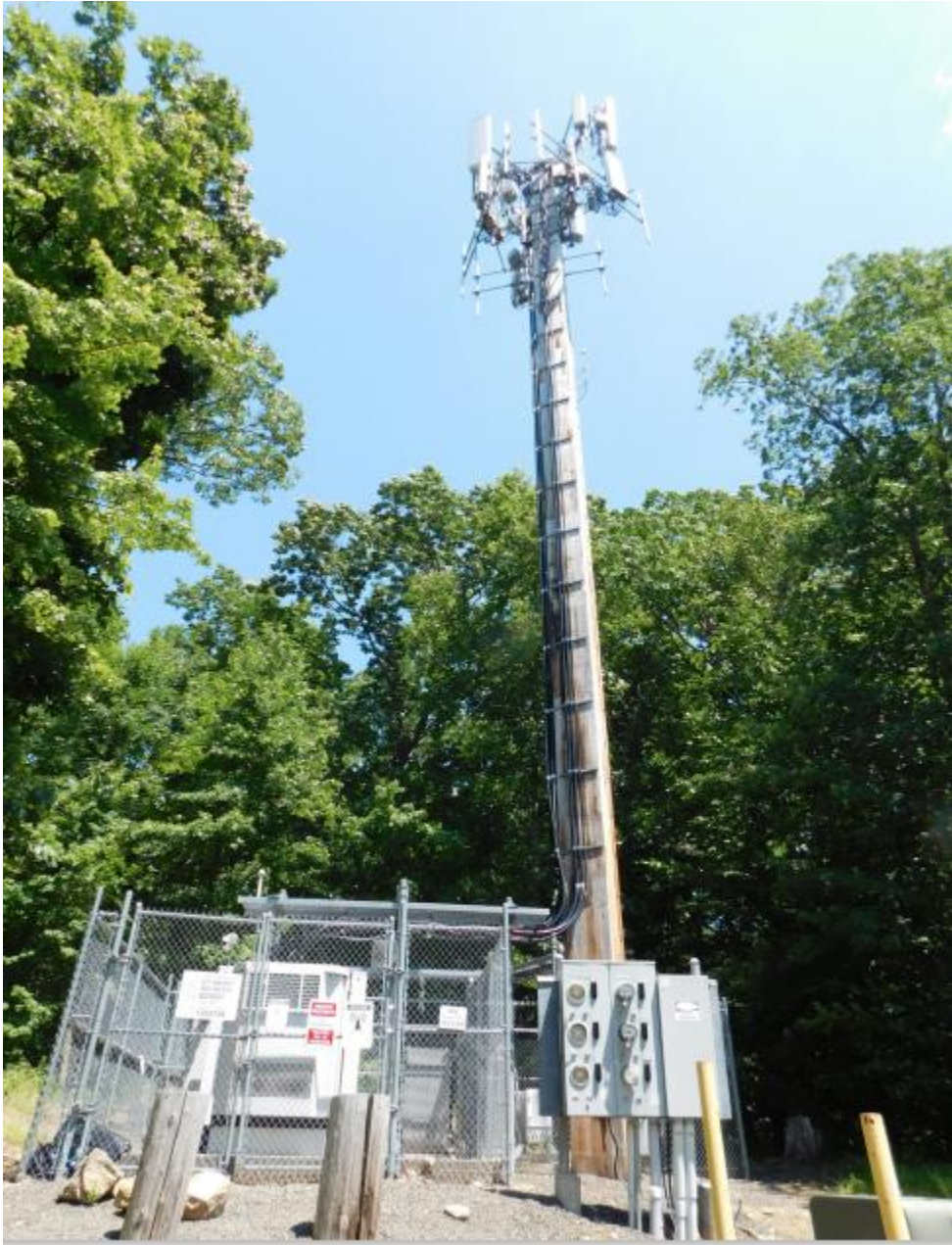
Figure 1 - Existing Laminate Wood Pole
