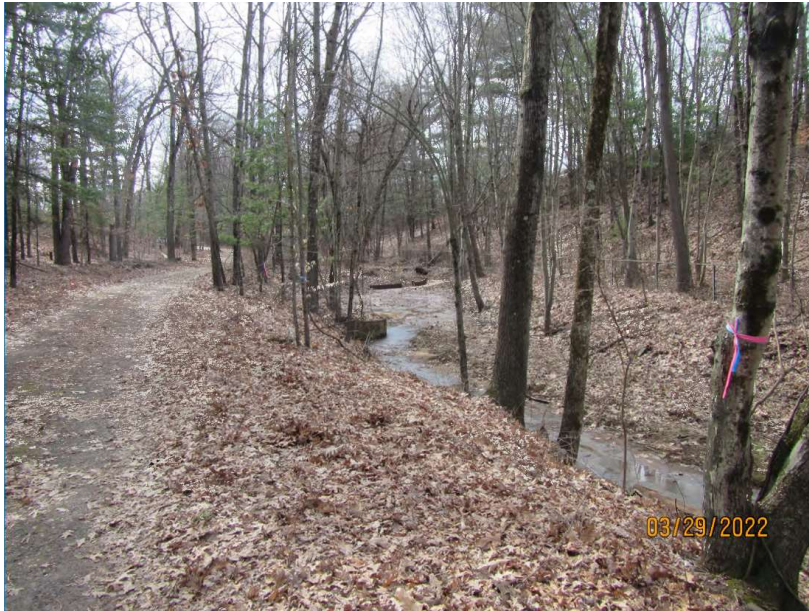
No. 5 - Photo of Wetland 2 taken at flag 100, facing southeast. A segment of Rainbow Brook was relocated to construct the Bradley Connector.
