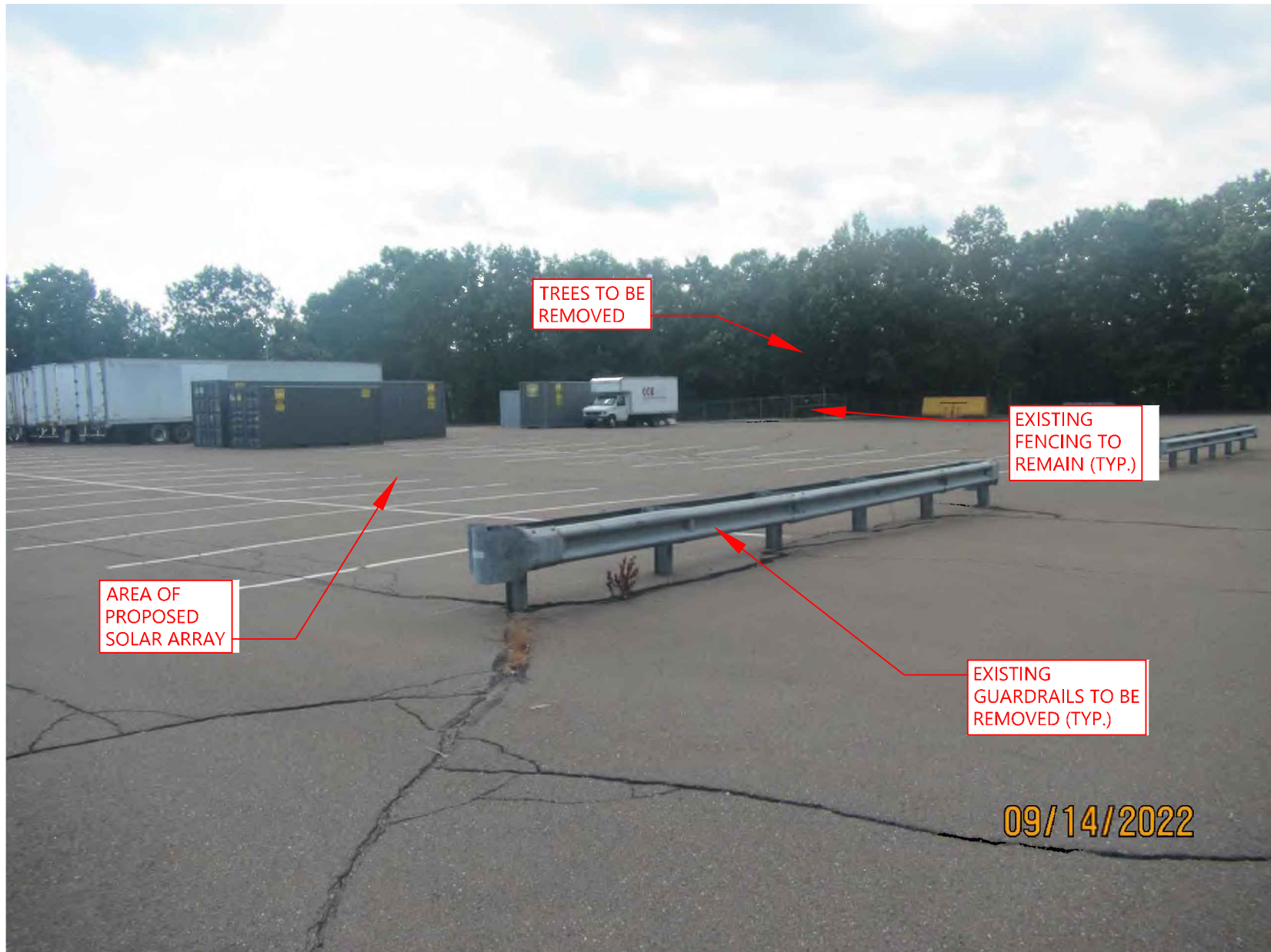
Photo 11 Existing Paved Project Area
