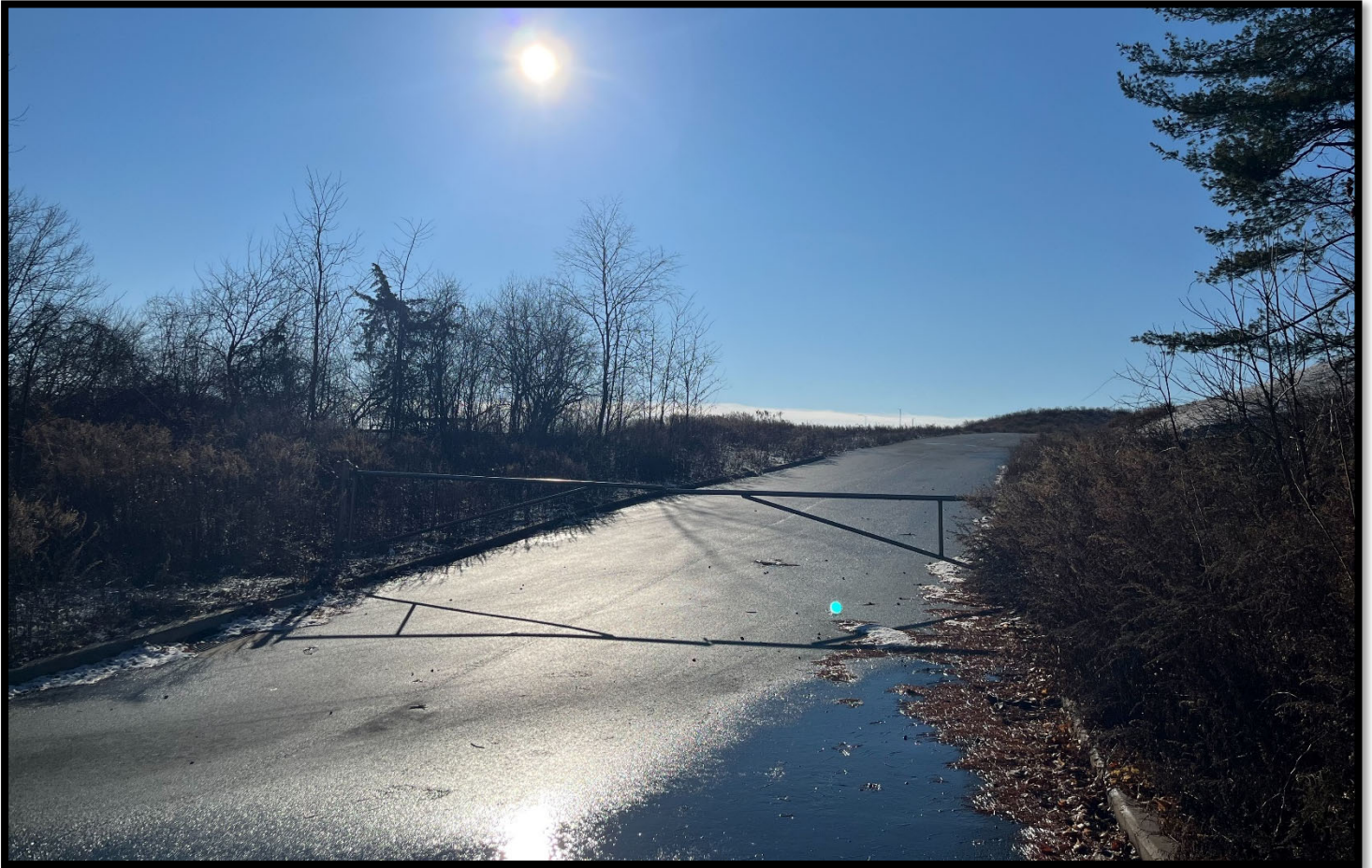
Photo #5 Description: Taken from Division Street looking south (roof not visible).
