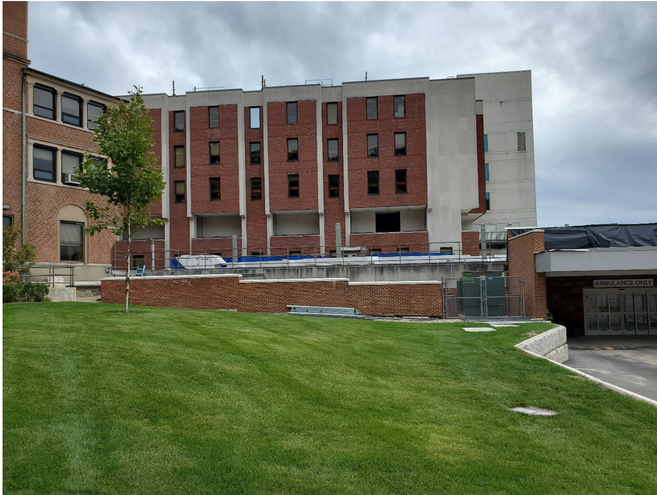
Looking toward Facility location; Hospital Emergency Department entrances to right
