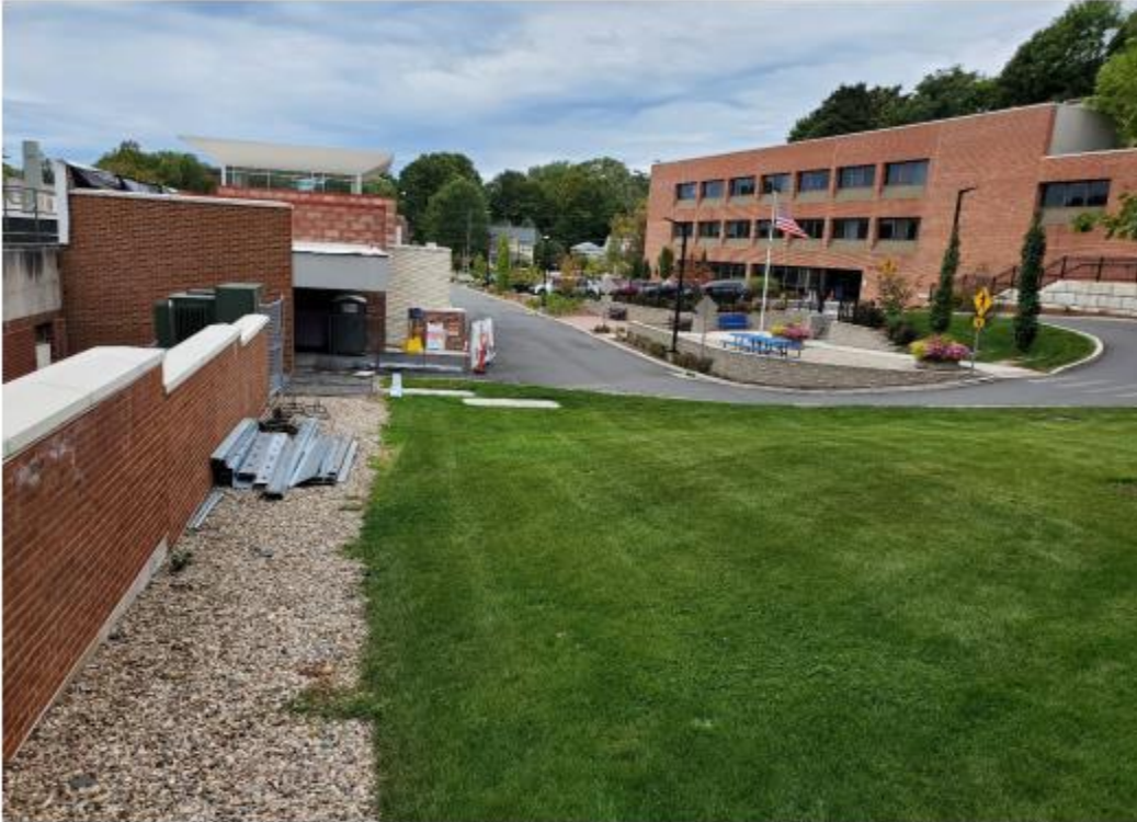
Looking west toward Goodwin Street; Facility location in foreground
