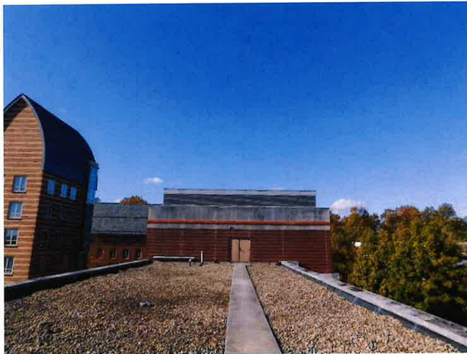
Photo 1: Sample photo illustrating the proposed location of the antenna enclosure (view from the East).
