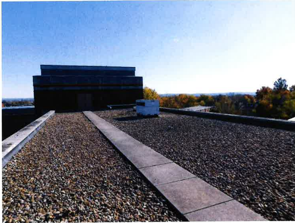
Photo 3: Sample photo illustrating the proposed location of the equipment platform (view from the West).
