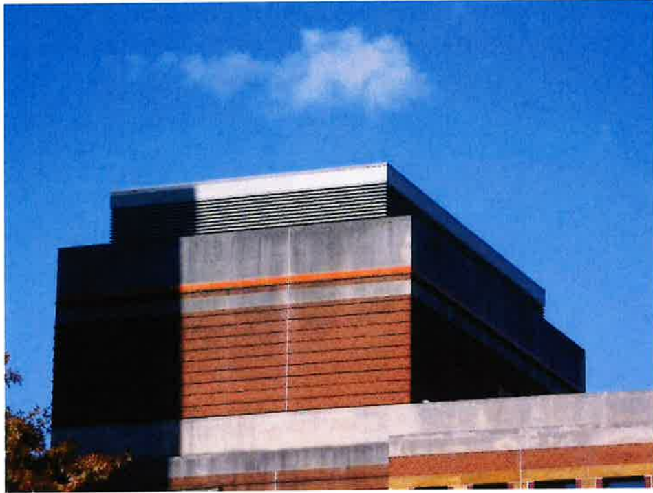
Photo 1: Sample photo illustrating the proposed location of the antenna enclosure (view from the South).
