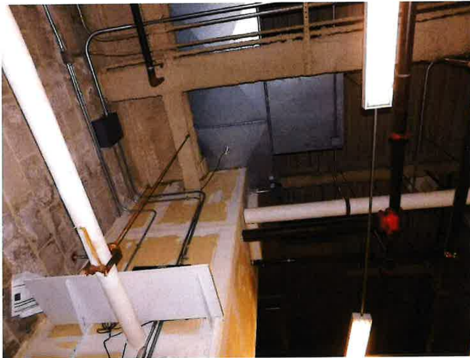
Photo 4: Sample photo illustrating the existing roof framing (fireproofed).
