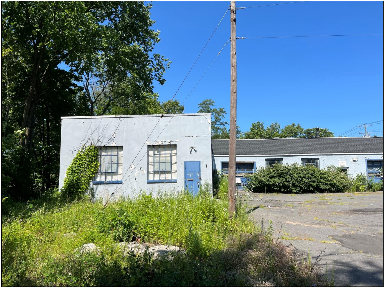
Photo 5. Detail photo of existing structure in project area, looking west.
