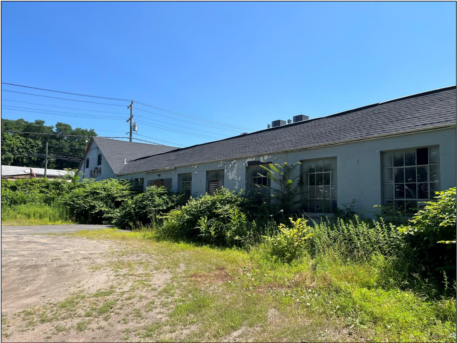
Photo 11. Detail photo of existing structure in project area looking northwest.
