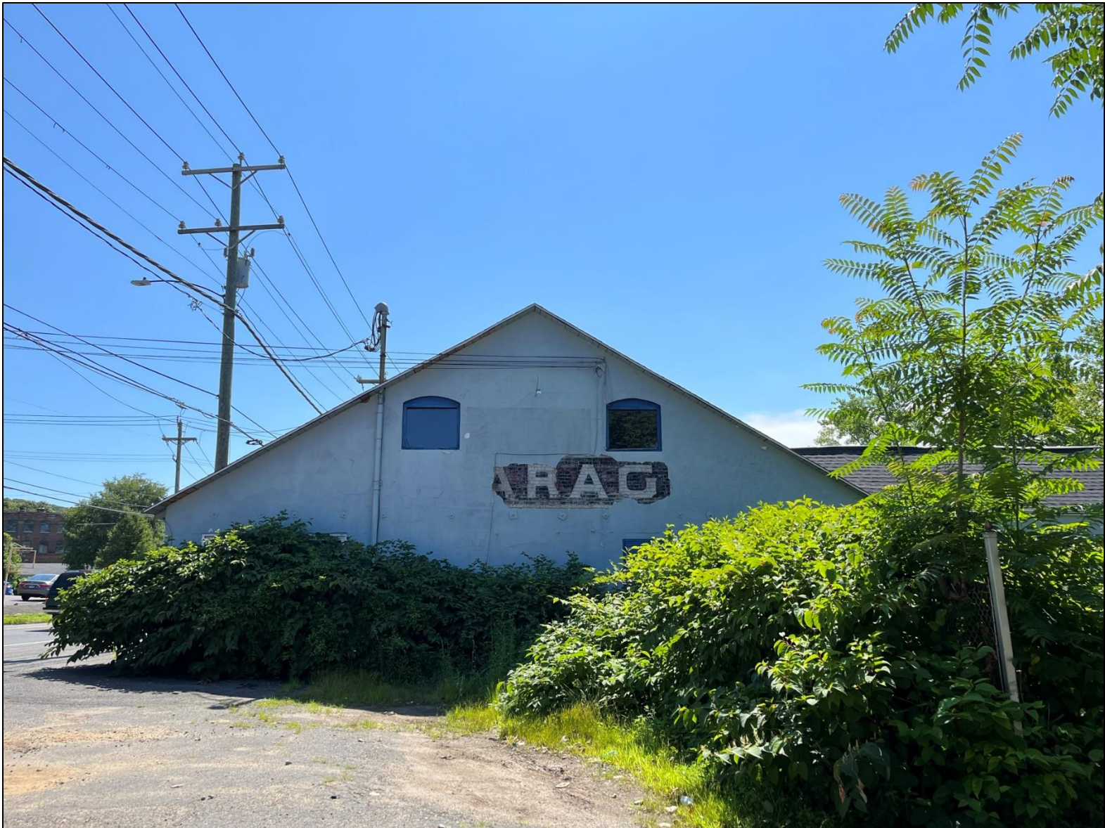
Photo 12. Detail photo of existing structure in project area looking east.
