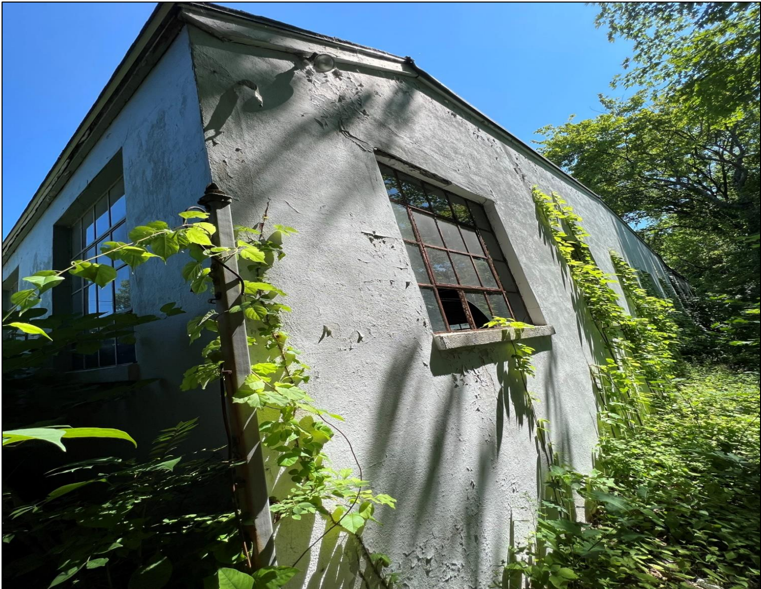
Photo 8. Detail photo of rear wall of existing structure in project area, looking northeast.
