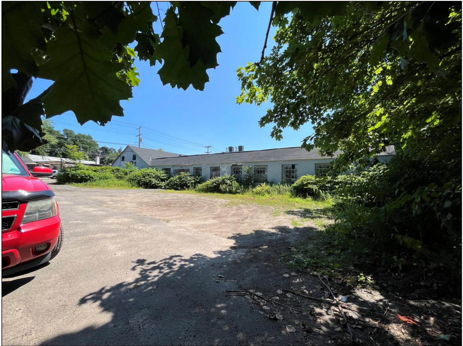
Photo 10. Overview photo of project area taken from rear edge of lot facing northeast.
