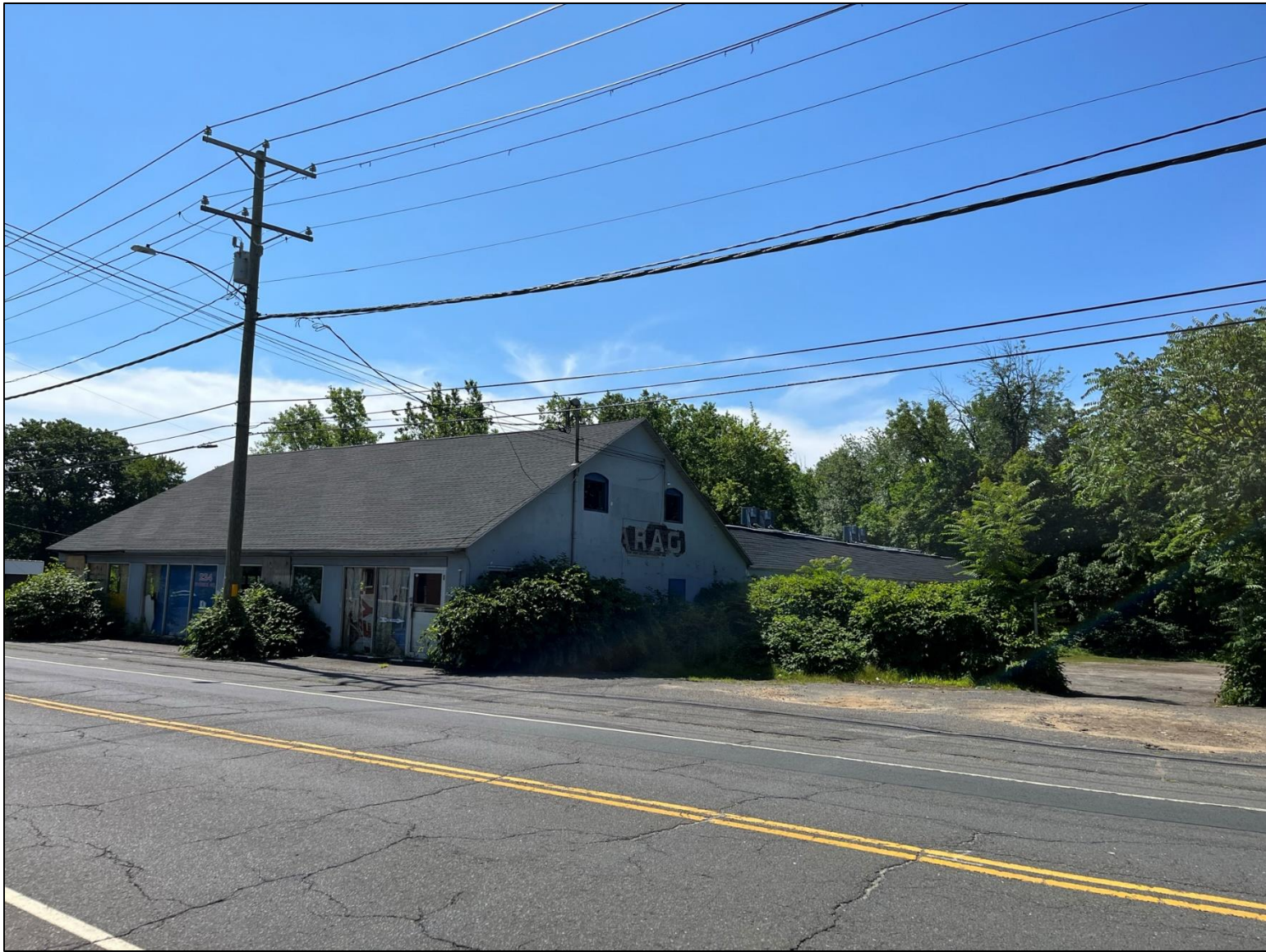
Photo 14. Overview photo of project area taken from across Riverside Avenue facing southeast.
