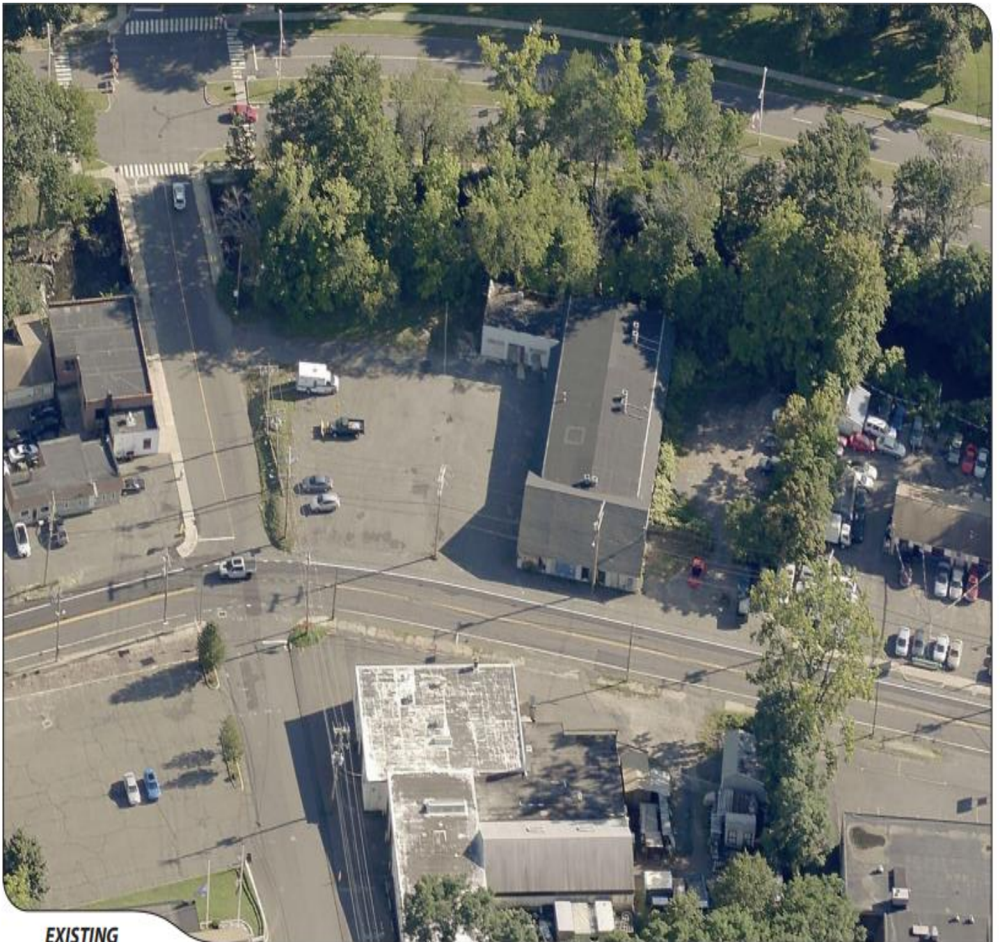
Figure 4: Existing Site Conditions
