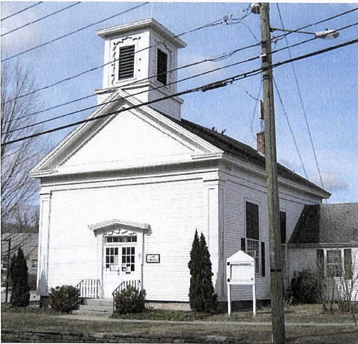
Photograph 2 of 5: CT_New London County_Lyme Town Hall_002 East elevation, looking west
