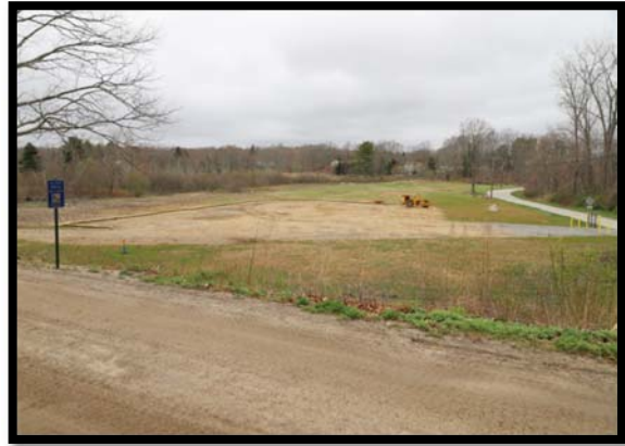
Figure 2: Site view from the Air Line Trail, Colchester Spur (West)
