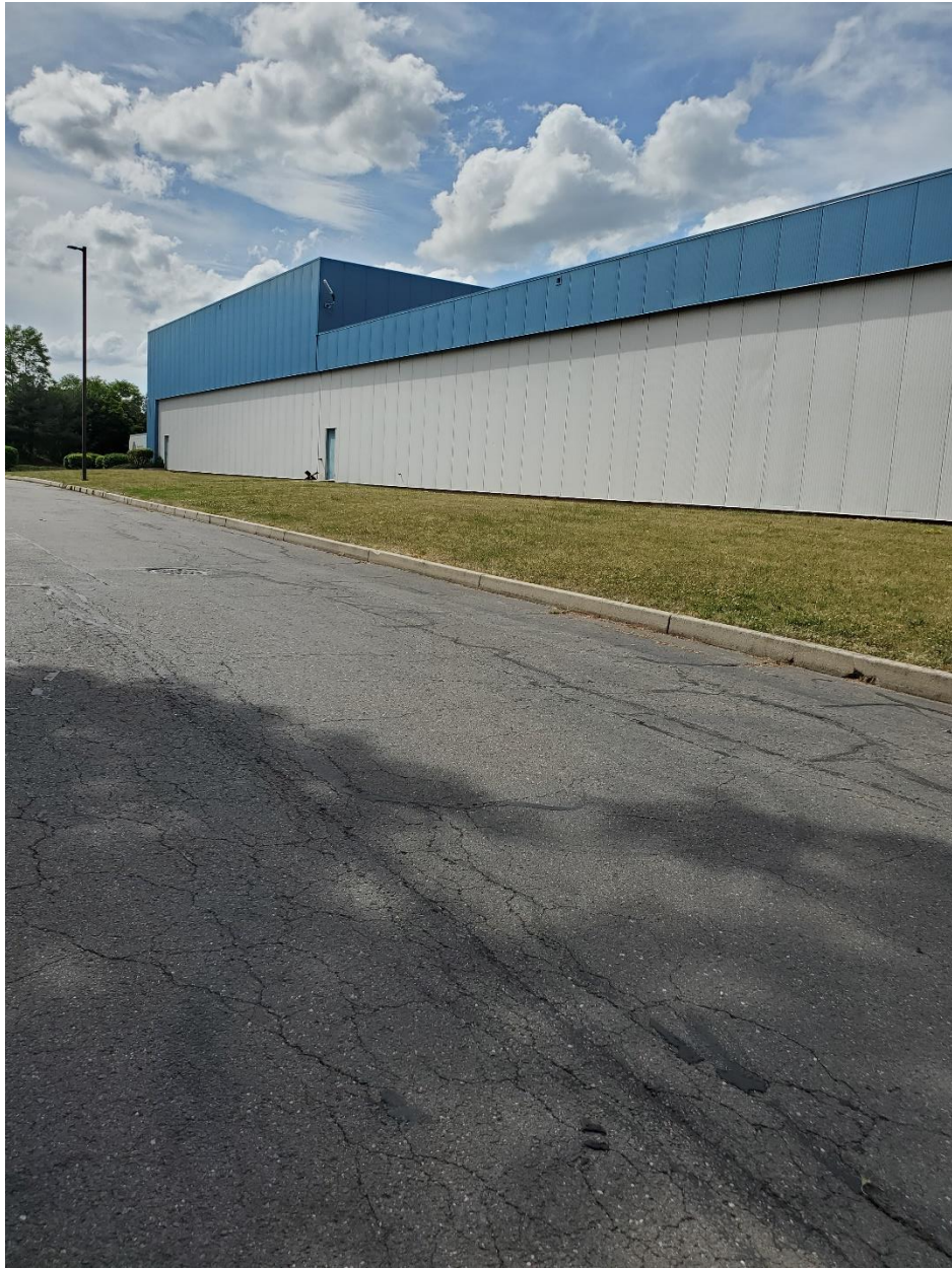
Looking northwest toward Facility location
