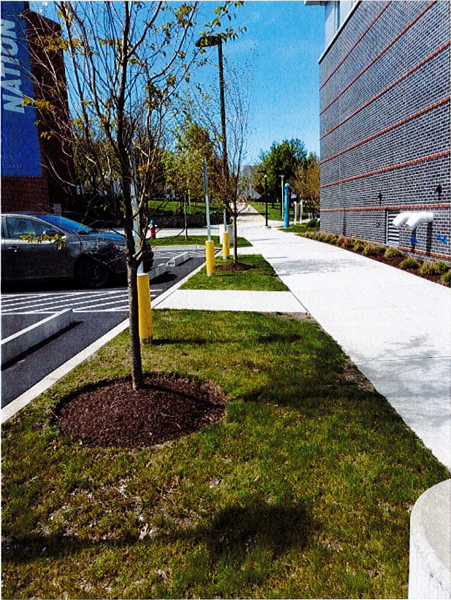
Looking north; Facility location at left
