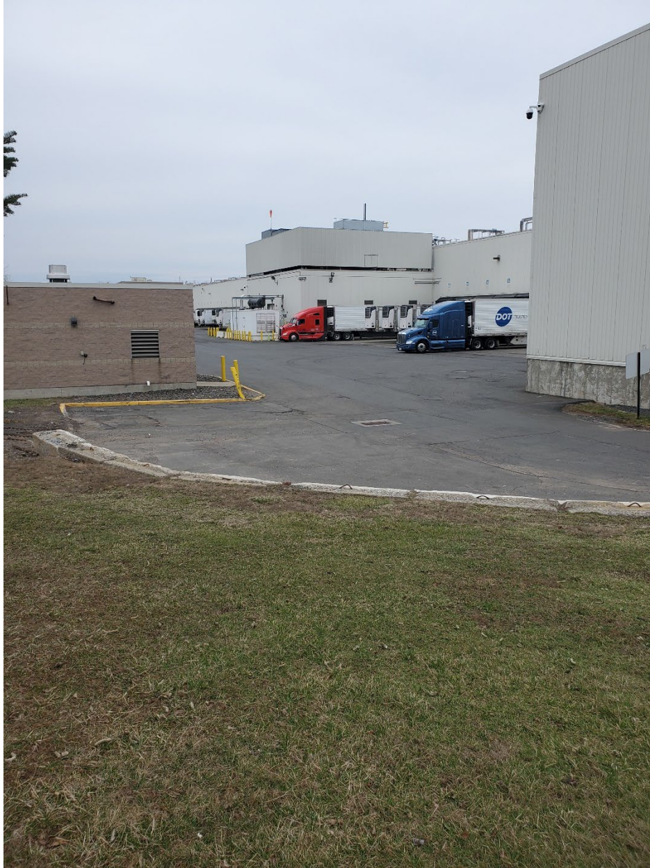
Looking north from along Industrial Avenue; Facility location behind "L" of Building B at center
