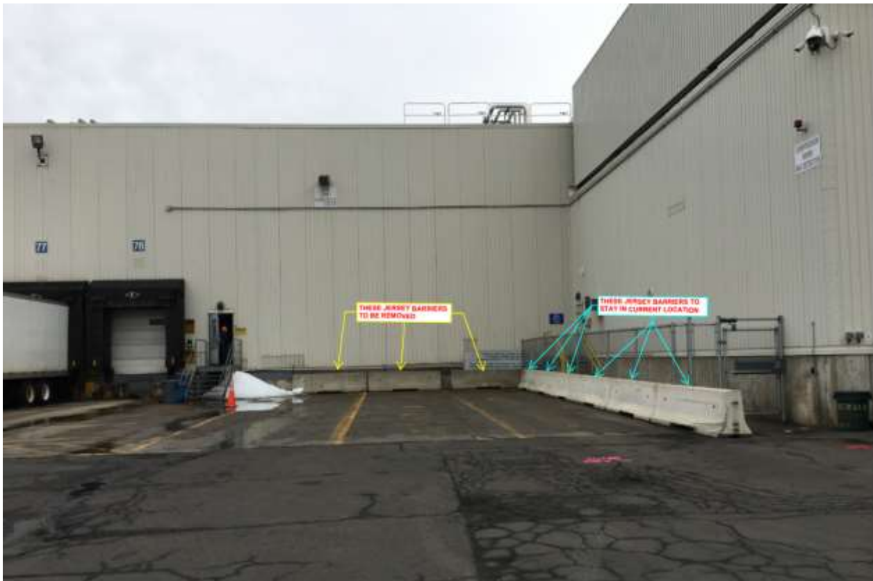
Looking east towards Facility location.
