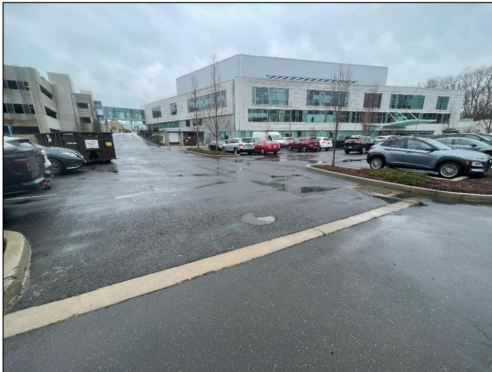
Photo 2. Overview photo of project area facing northwest.
