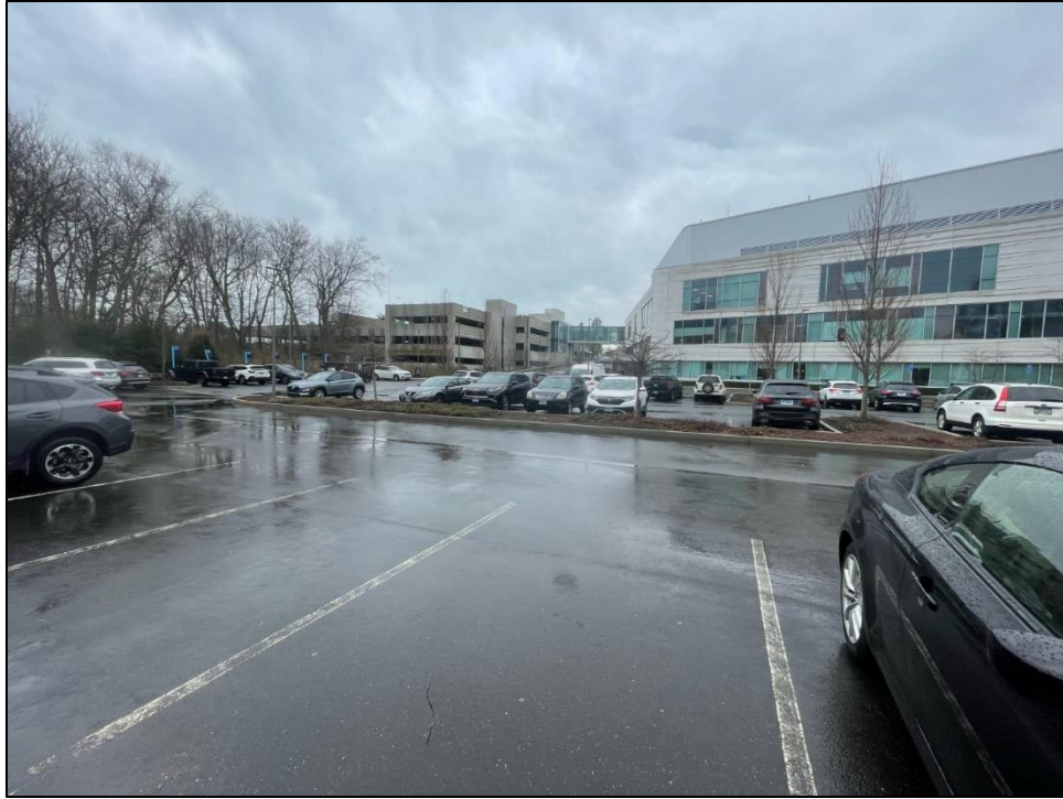
Photo 2. Overview photo of location of the fuel cell facing west.
