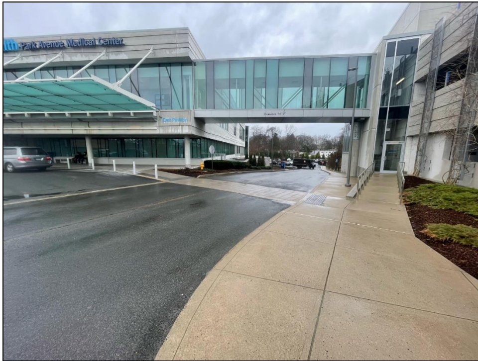
Photo 1. Overview photo of the location of proposed buried utilities facing east.
