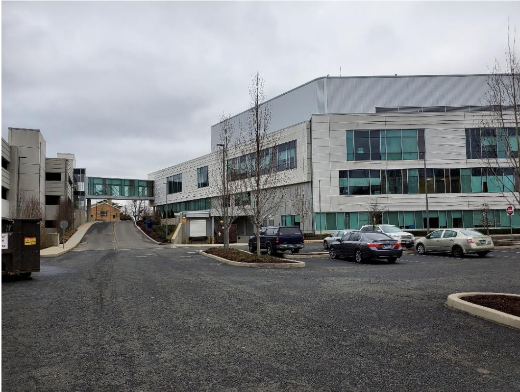
Looking west toward Facility location at center of photo (to right of trees); building in background.
