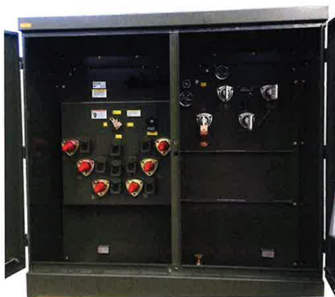
Fig 2. Three Phase Maddox Padmount Transformer
