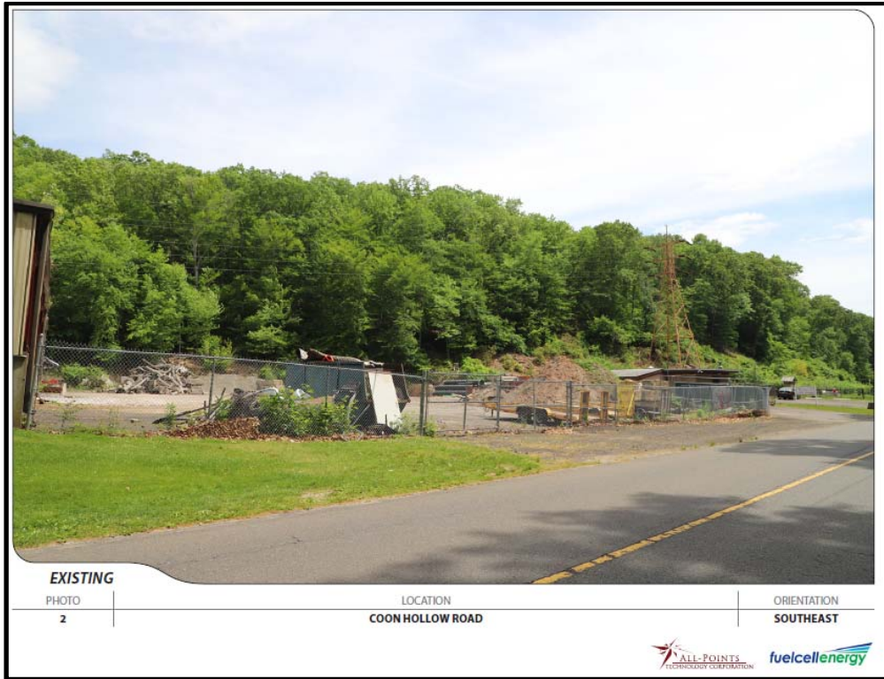
Figure A5 Existing Site Condition– Roadside From Coon Hollow Rd. and Looking Southeast
