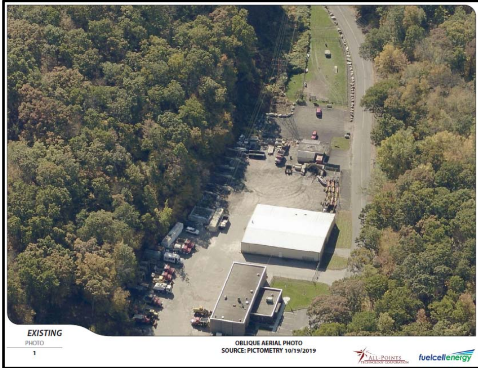
Figure A3 Existing Site Conditions– Looking South at Coon Hollow Rd.
