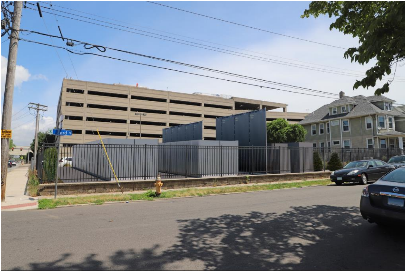
Landscaping and “Acoustiblock” sound barrier shown.
