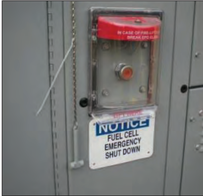
Figure 1: Emergency Power Off Button
