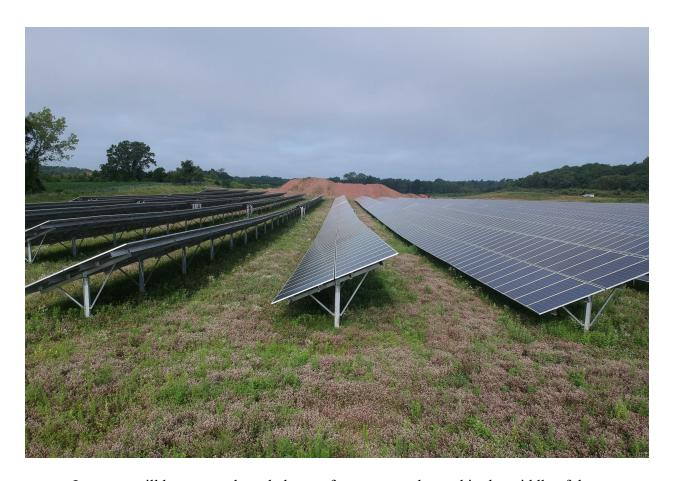
Inverters will be mounted at a balance of system area located in the middle of the array, where small concrete pads will also be installed for transformers and switchgears. Construction of the Project will require 7.33 acres of tree clearing with a total development area of 11.6 acres. At the end of the operational life of the Project, Lodestar will remove all equipment (*e.g.* racking system, panels, inverters, electrical collection system, equipment pads, etc.) from the Project Site.
