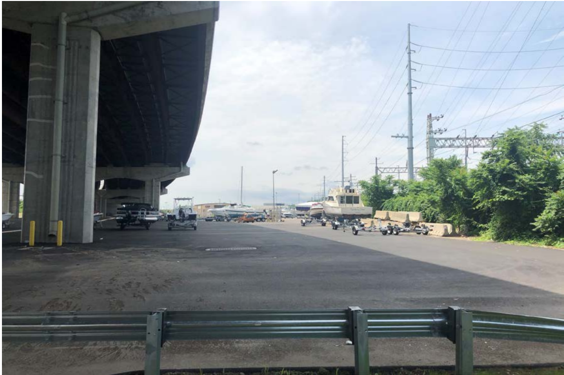
Photo 1: View of proposed tower and compound by boat and jersey barriers in right side of photo at pavement edge, looking west. I-95 Housatonic Bridge in left side of photo and Metro North railroad in far right side of photo.
