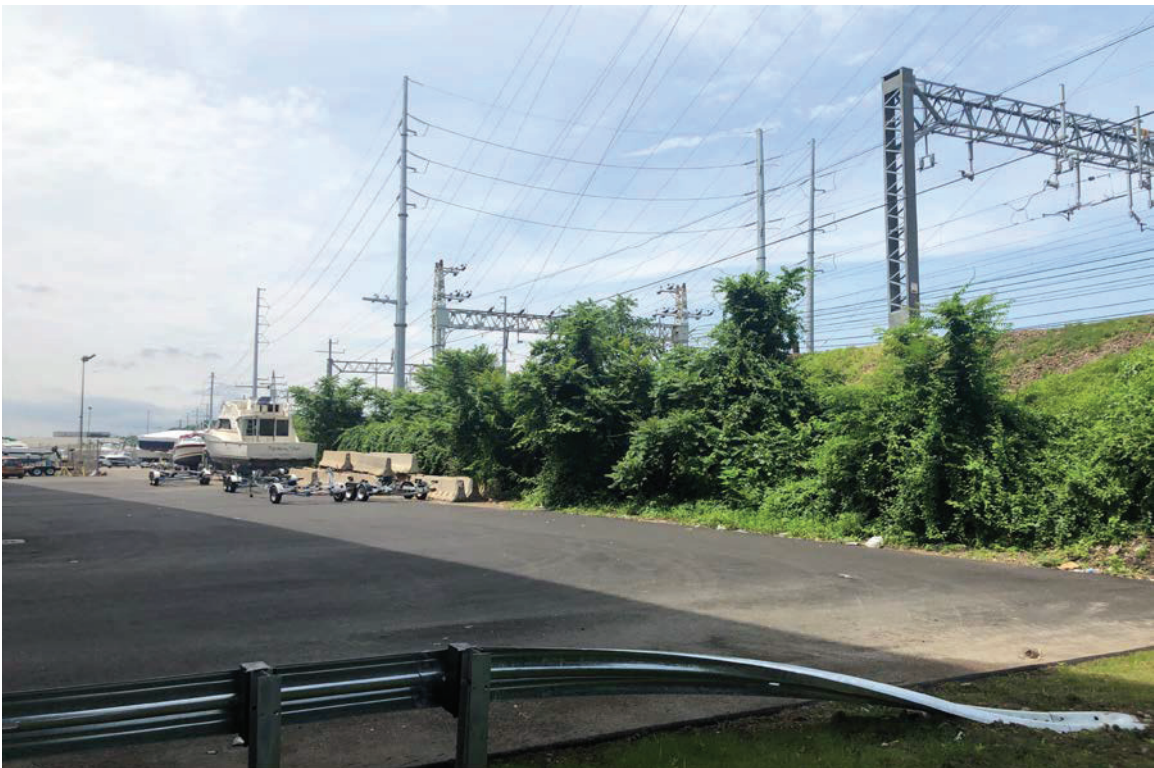
Photo 2: View of proposed tower and compound (elevated compound along rip rap armored side slope) looking west.
