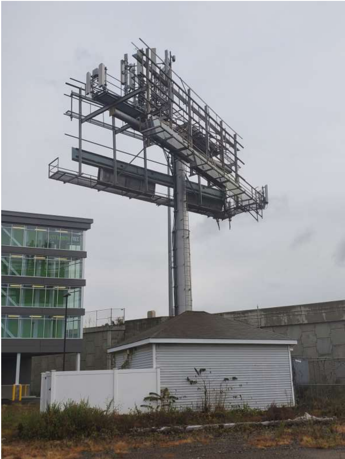
Figure 2. Existing NTAA Structure at 28 Sidney Street.
