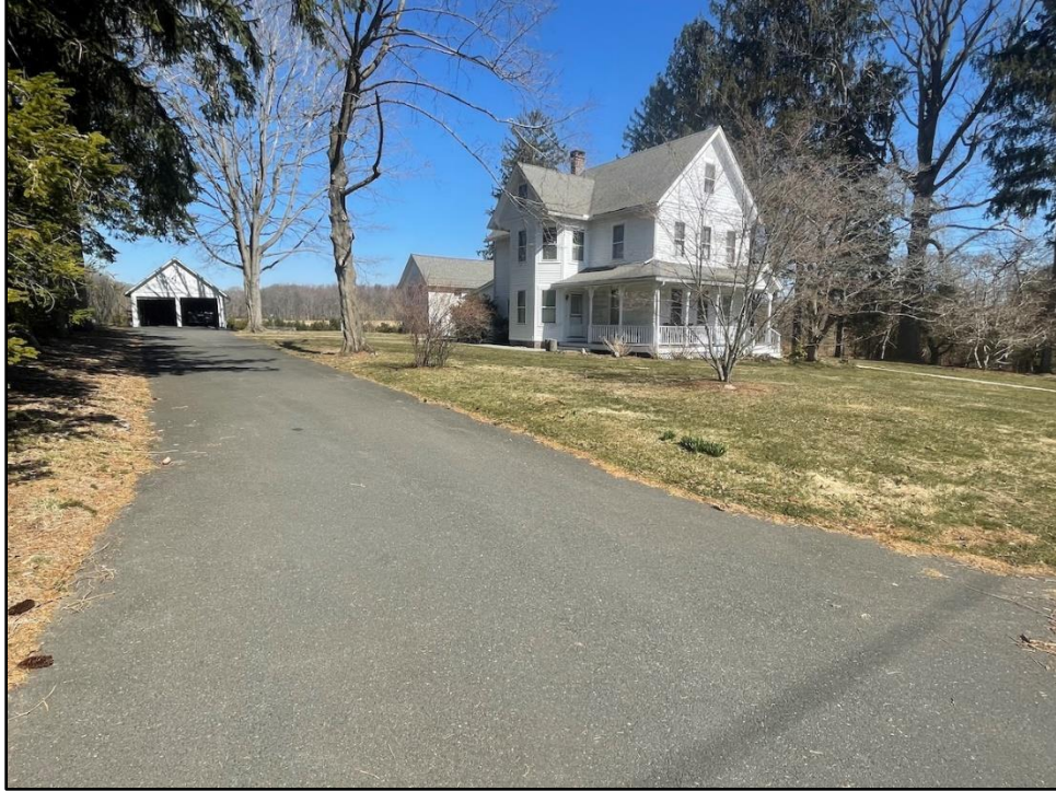
Photo 29. Overview of 353 Old Tavern Road facing northeast.
