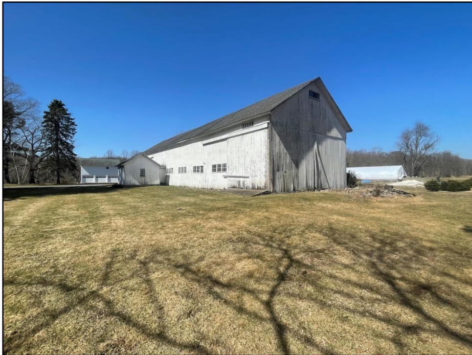
Photo 30. Overview of the Treat Farm English barn, listed on the State Register of Historic Places, facing northwest.
