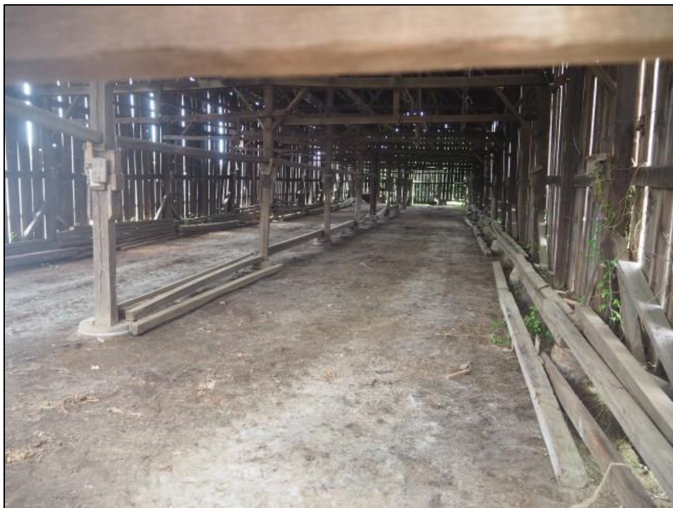
Figure 44. Interior view of Tobacco Shed No. 4 looking northwest.
