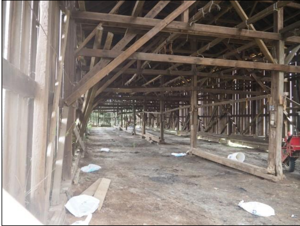
Figure 43. Interior view of Tobacco Shed No. 1 looking west.
