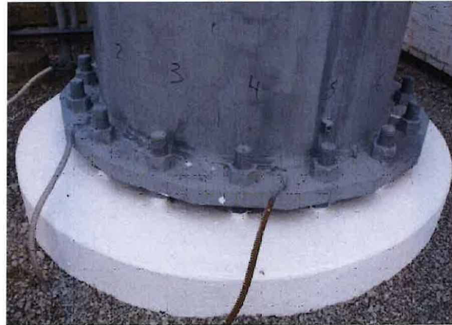
EXAMPLE OF FOUNDATION COATING (REFERENCE ONLY)
