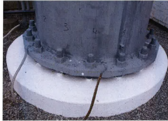
EXAMPLE OF FOUNDATION COATING (REFERENCE ONLY)
