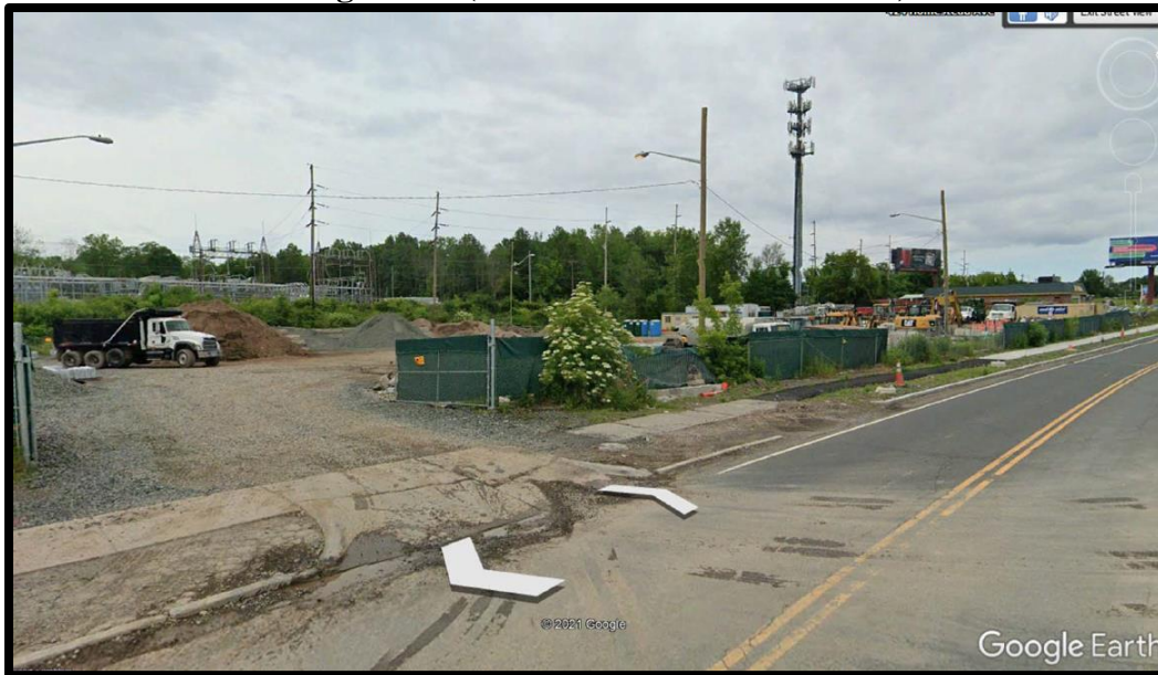
Figure 2B (View from Southeast of Site)
