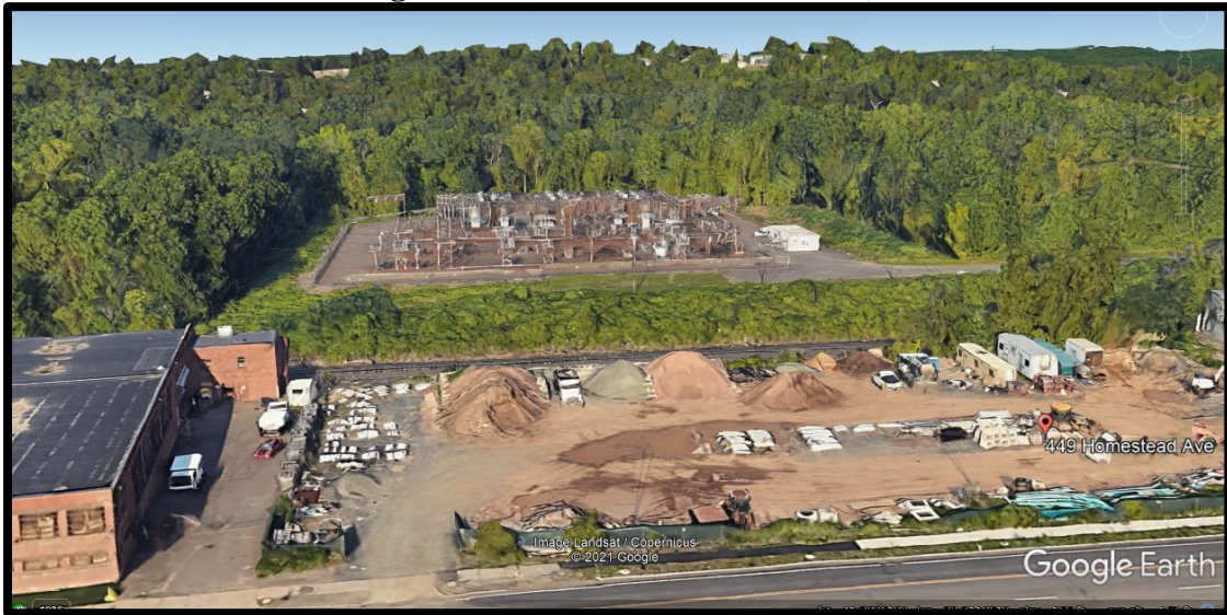
Figure 2A (View from East of Site)
