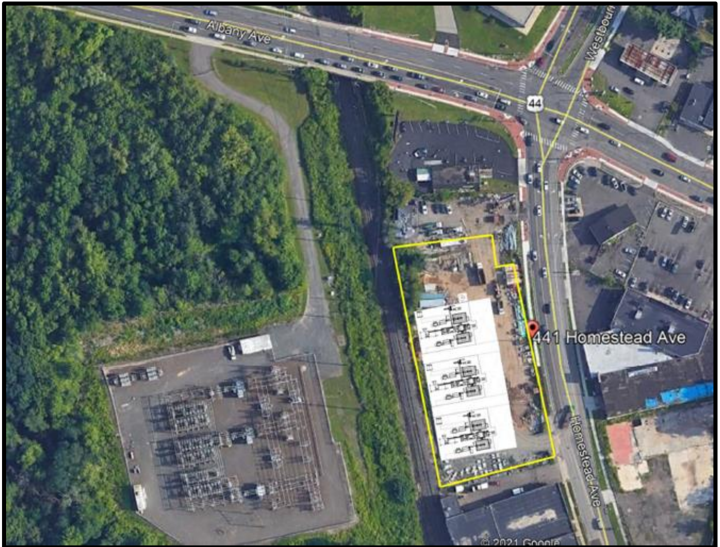
Aerial map of proposed Project area and approximation of three fuel cell systems.
