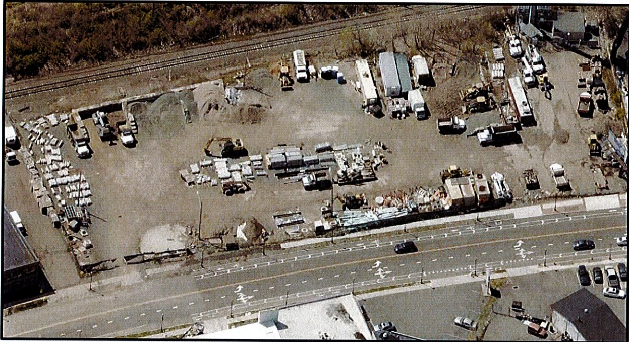
Figure 4. Existing Site conditions
