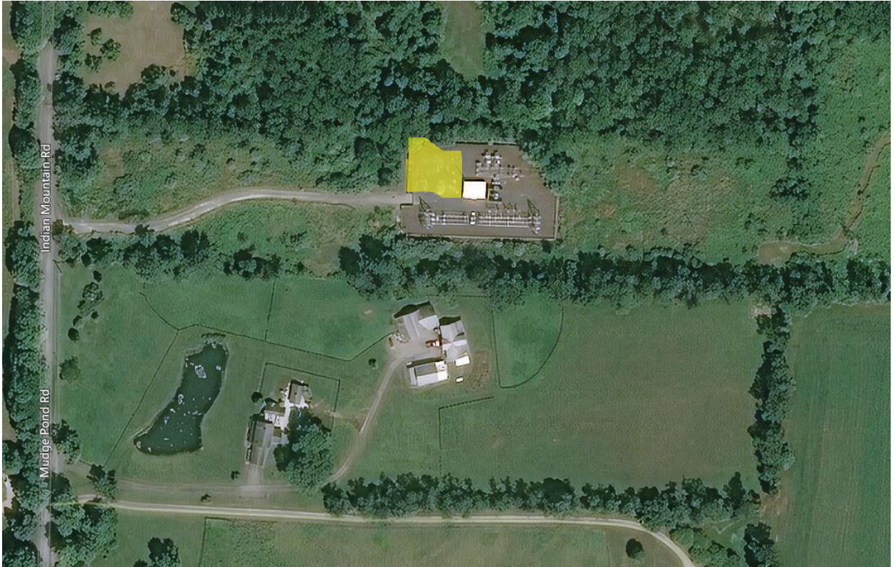
Figure 4 – Salisbury Substation Overview
