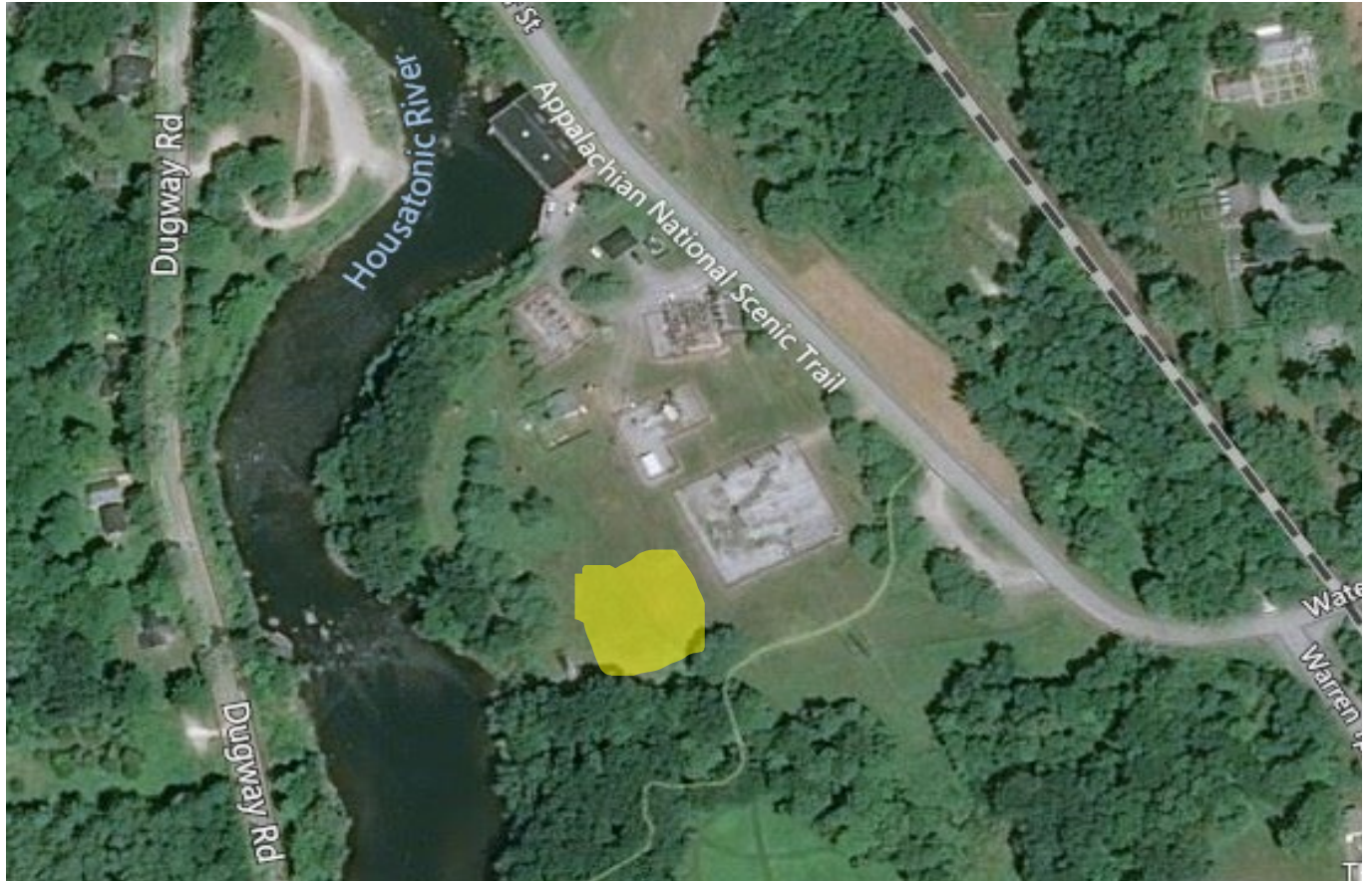
Figure 3 – Falls Village Substation Overview
