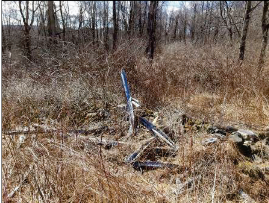
Photograph 7. Metal debris located on the boundary of the East Central Parcel and the Northeast Parcel, view toward the west
