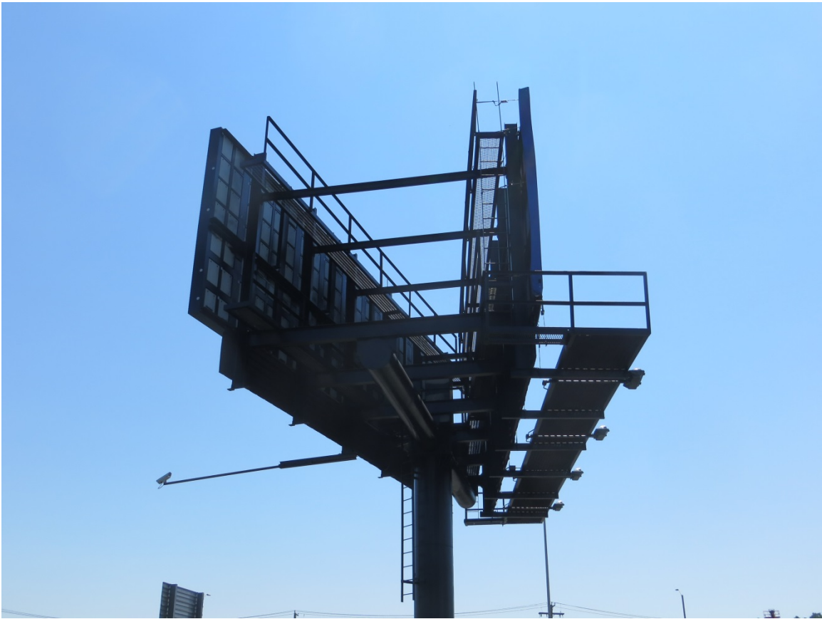
Photo 1: Photo illustrating the monopole with Appurtenances shown.
