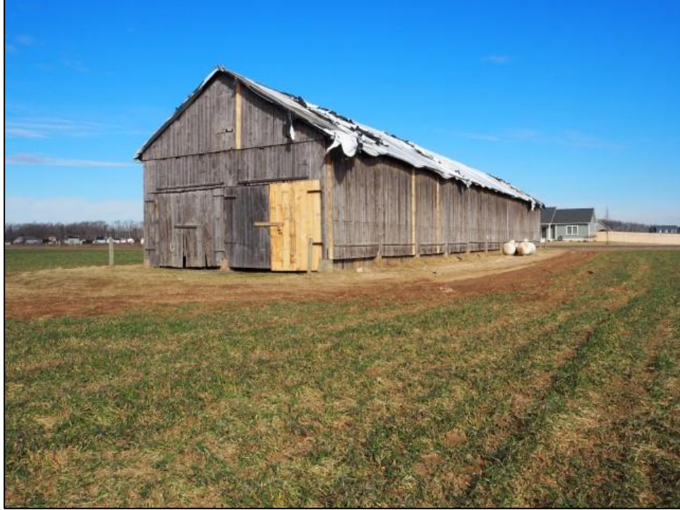
Figure 15. Photo of the tobacco shed near the development are facing northwest.
