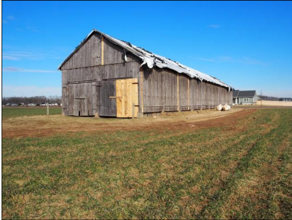
Figure 16. Photo of the tobacco shed near the development area facing northwest.
